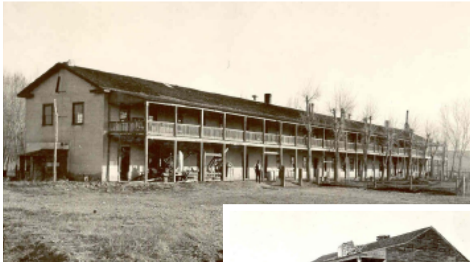
Old Fort Laramie Cavalry Barracks, 1909 Construction Photograph Albums, 1903-66 Office of the Chief Engineer RG 115, Records of the Bureau of Reclamation NARA-Rocky Mountain Region, Denver
