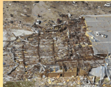
Figures 4 and 5. Damage in Dumas.
