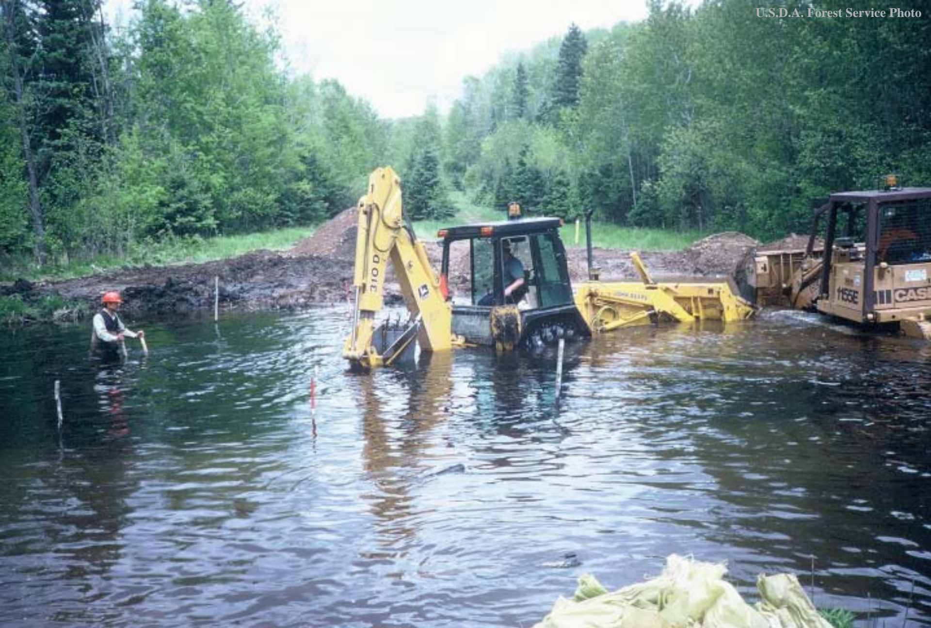
Pipeline Bridge Installation - Dozer and Backhoe in River
