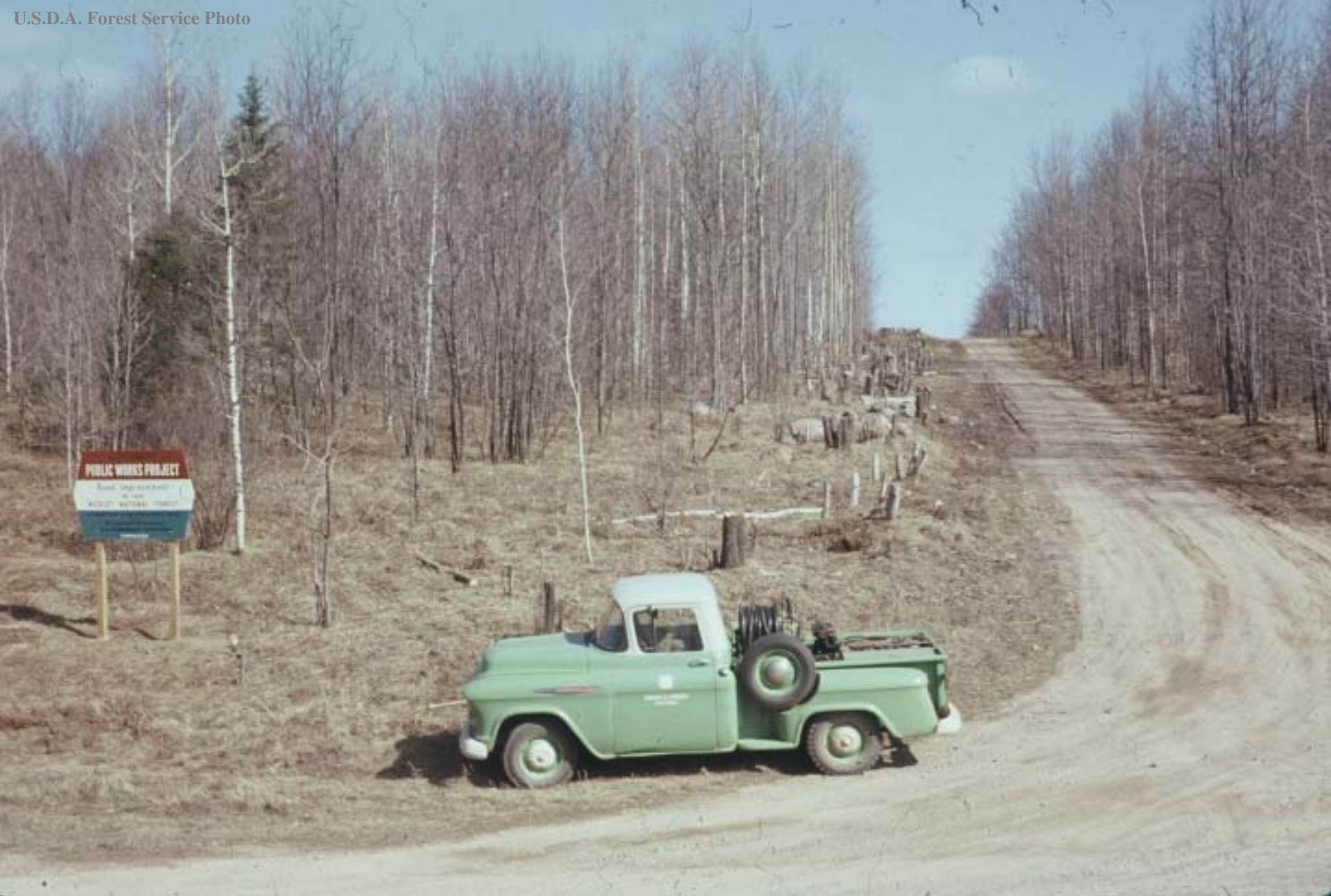
Boulder Lake Road (FR 2116) Construction, April 1963
