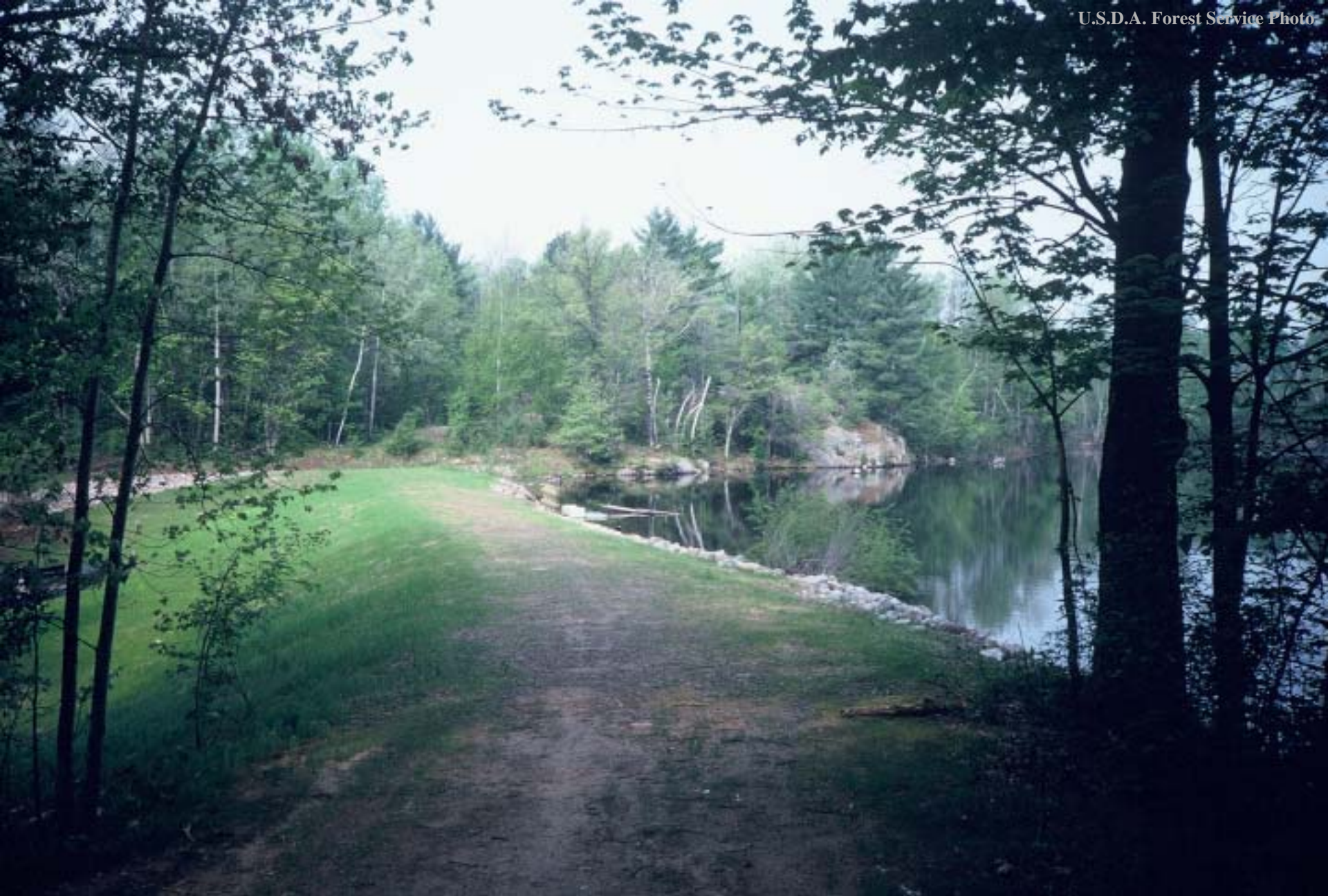
Waupee Dam After Reconstruction
