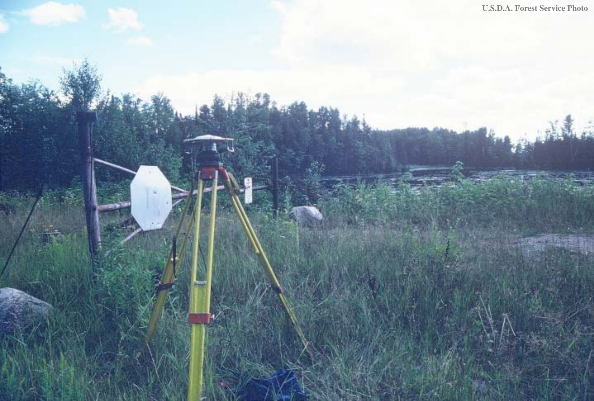
Surveying the Bluegill - Pickerel Lake Dam
