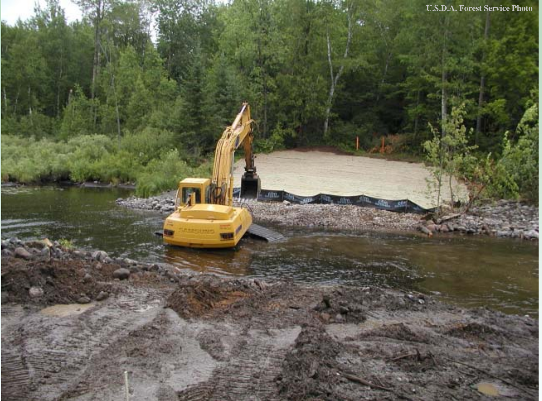
Hemlock Dam Removal – Excavator in River
