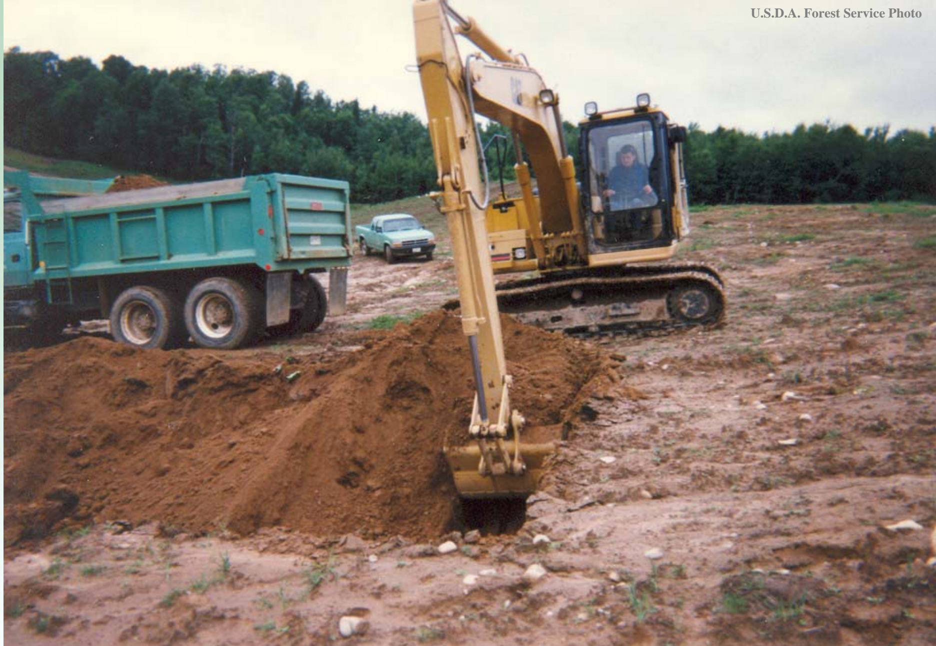
C&M Crew Excavating Silt for Lakewood Landfill
