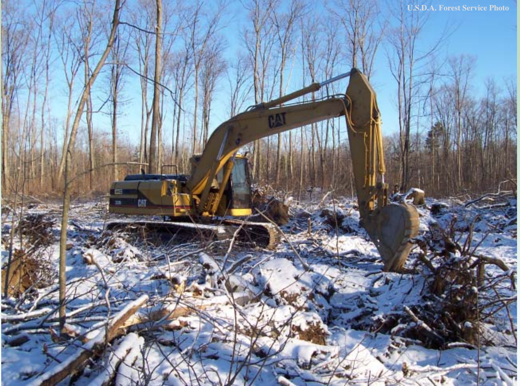
Excavator with Shovel Head Removing Stump Root Wads
