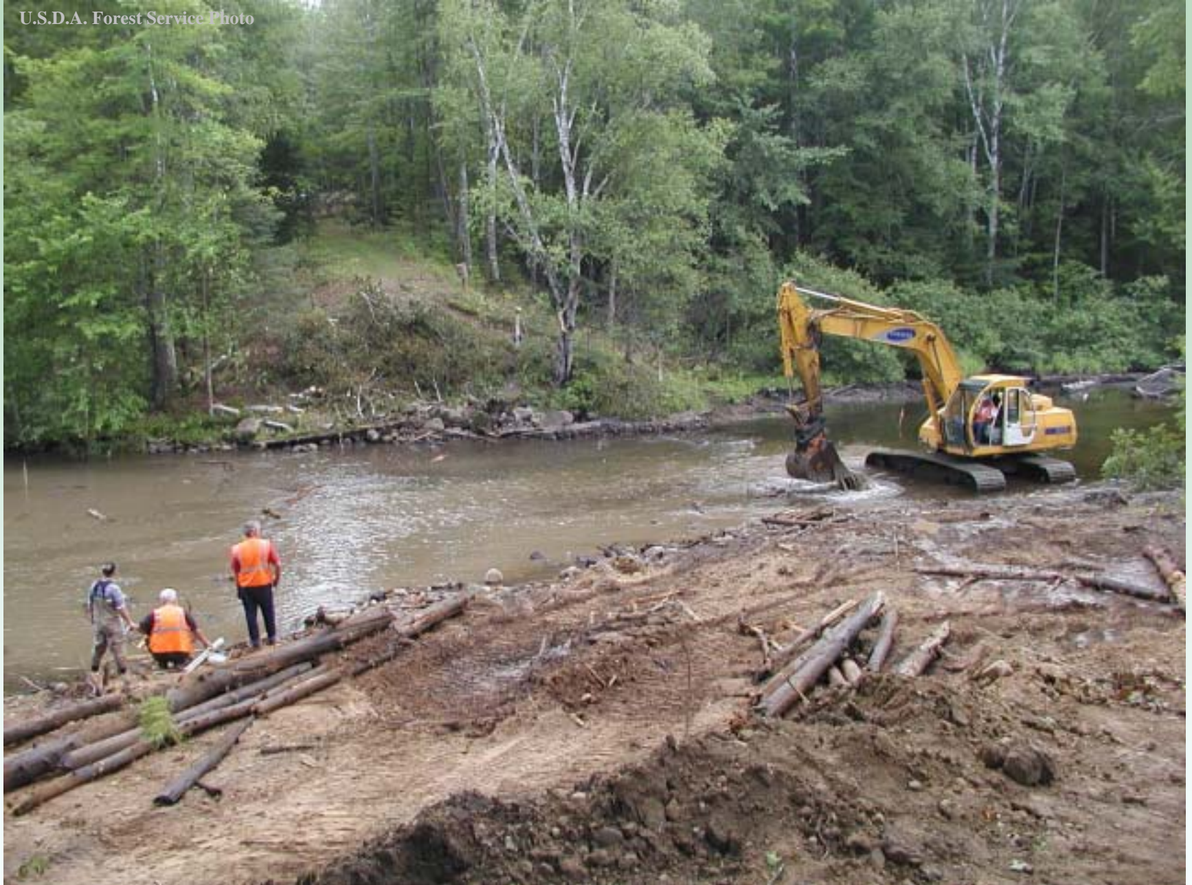
Knowles Dam Removal, Summer 2004
