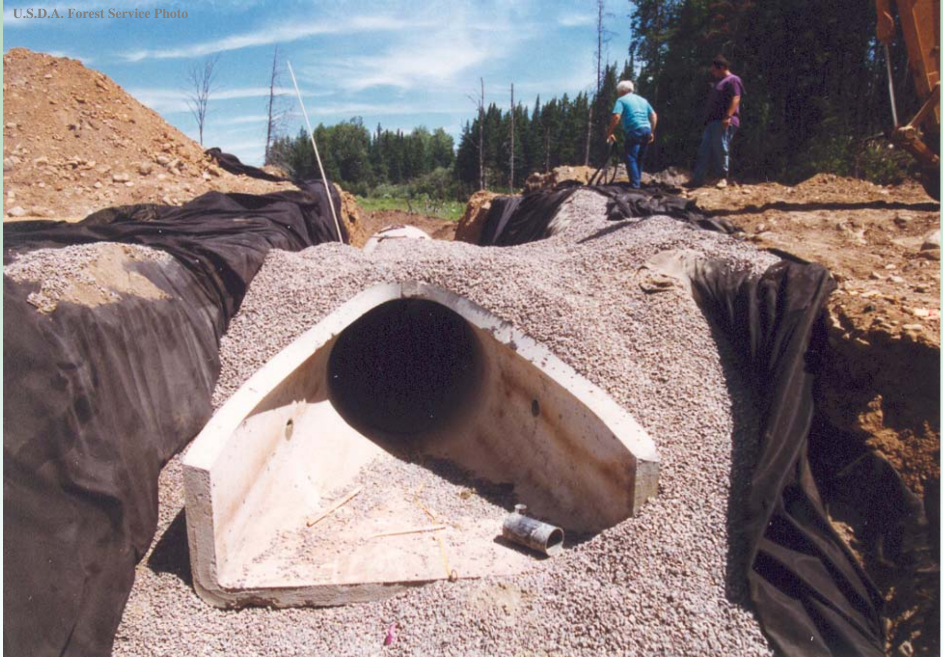
Washed Stone Around Pipe
