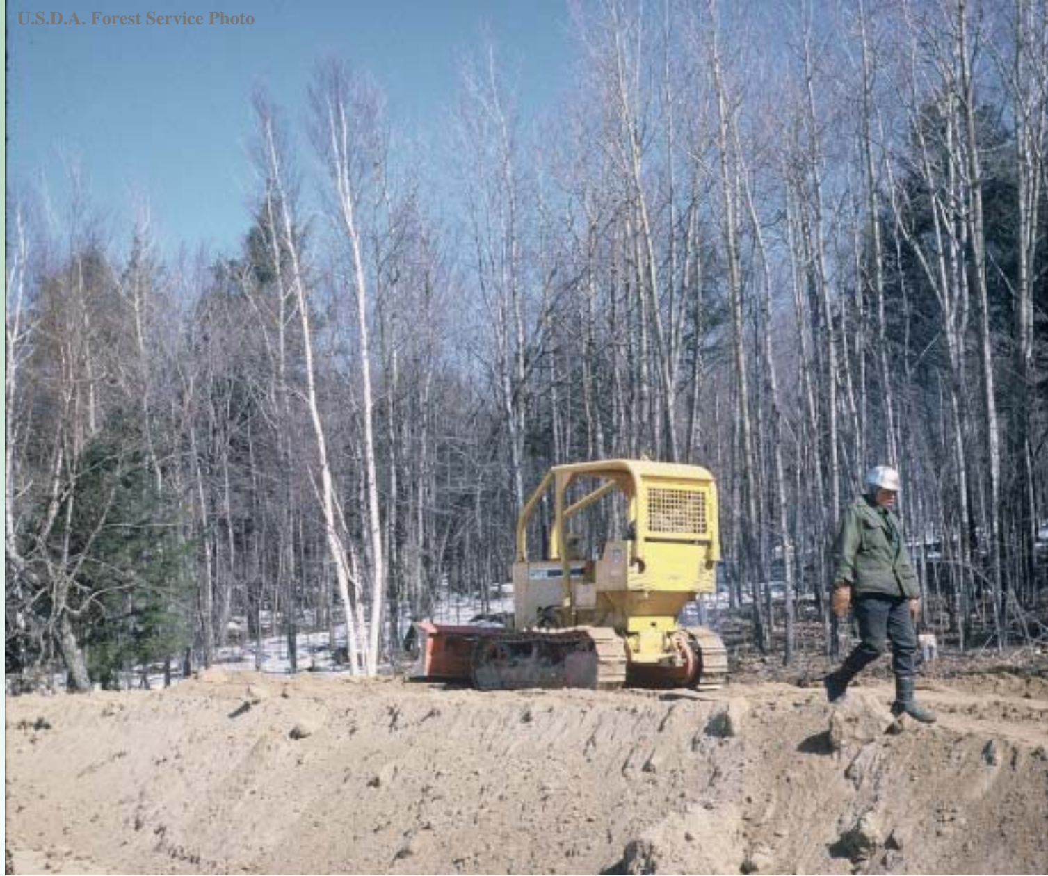
Blackwell Job Corps Constructing Ada Lake Campground, April 1968
