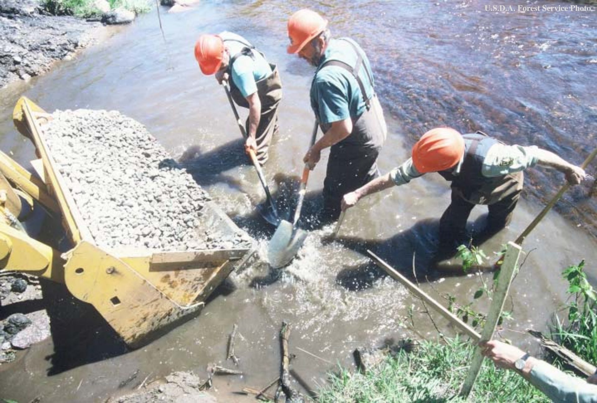
North Fork Thunder River Bridge Work
