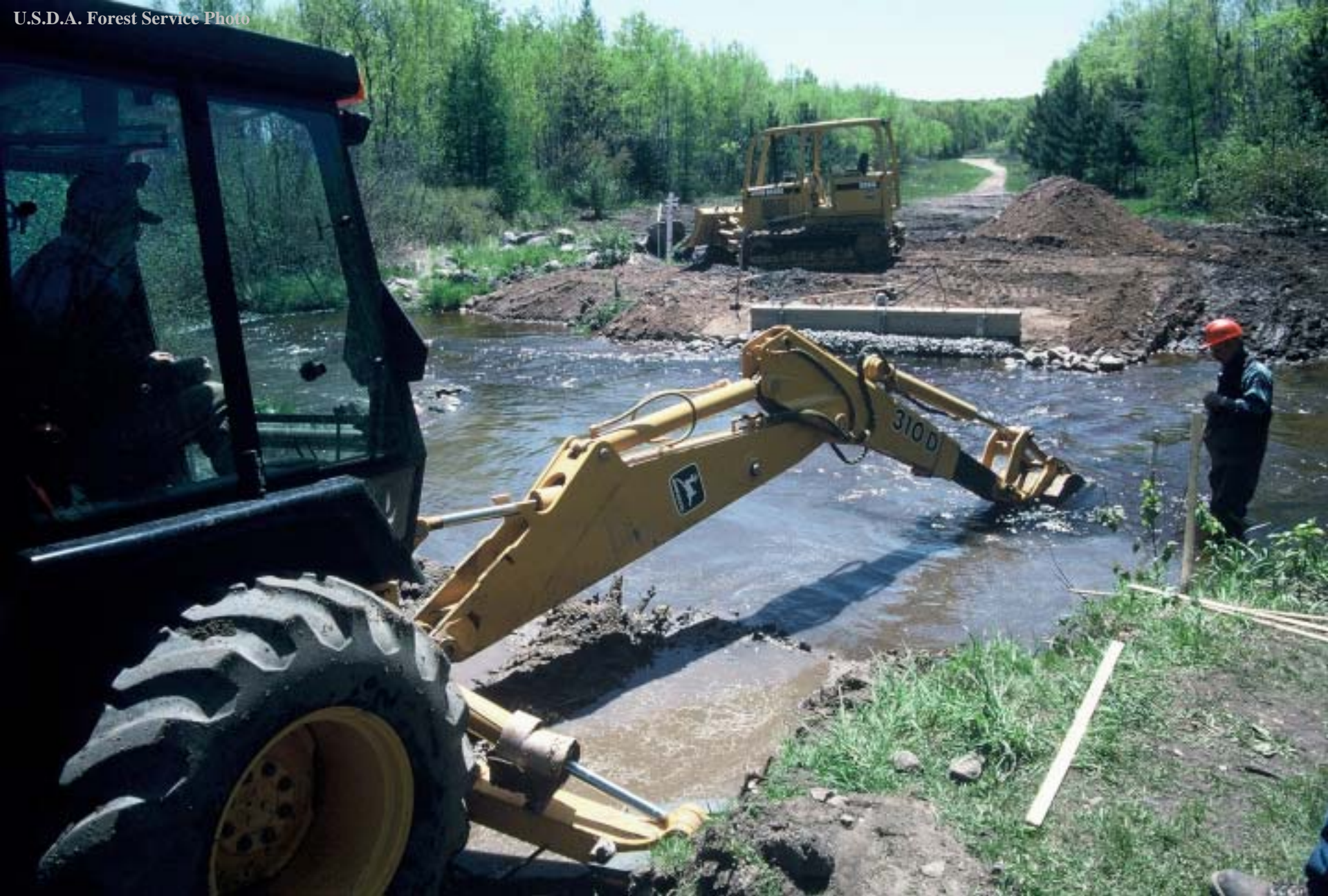
North Fork Thunder River Bridge Work
