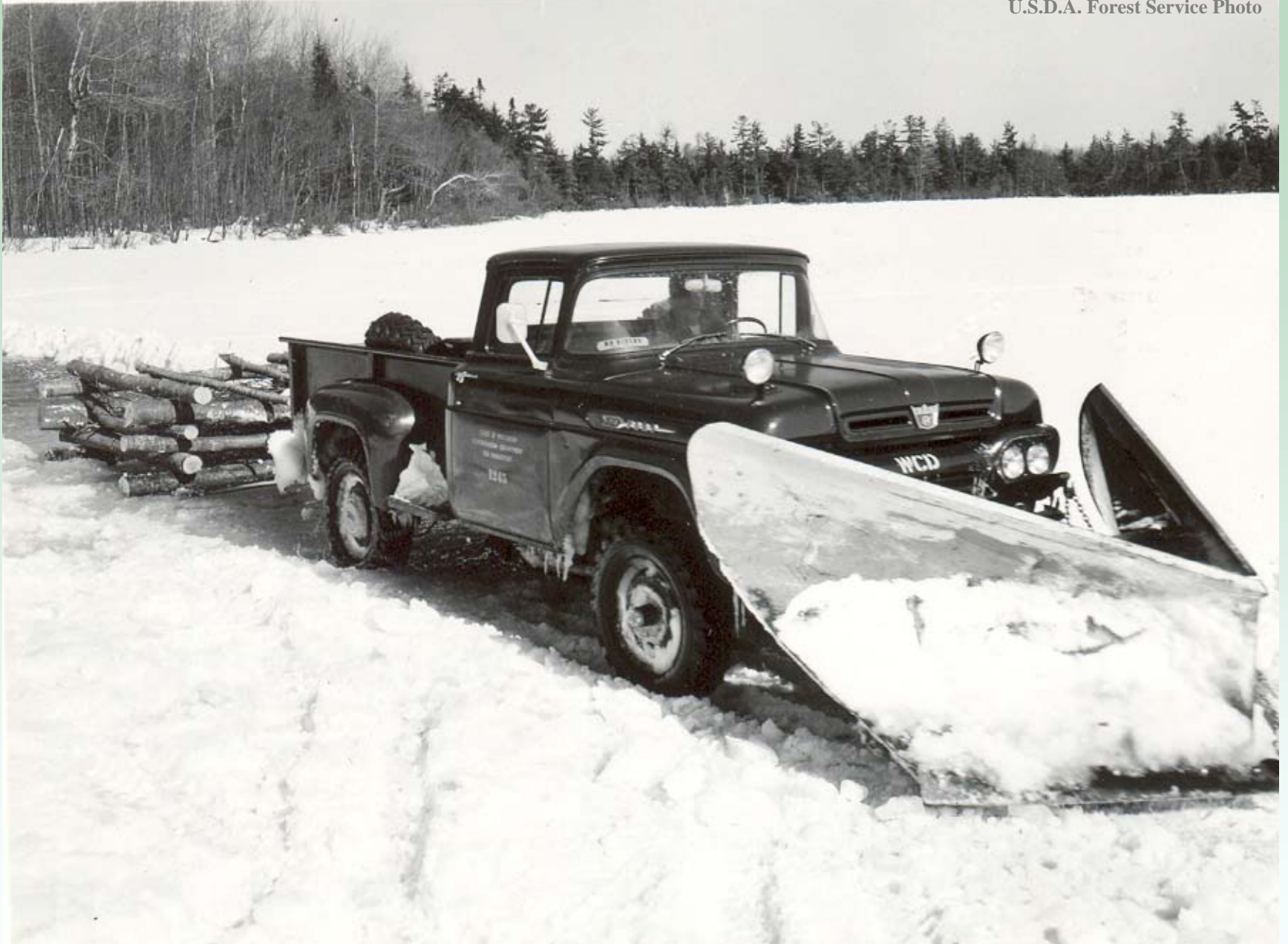
WCD Truck Towing Shelter onto Ada Lake Ice, February 1963
