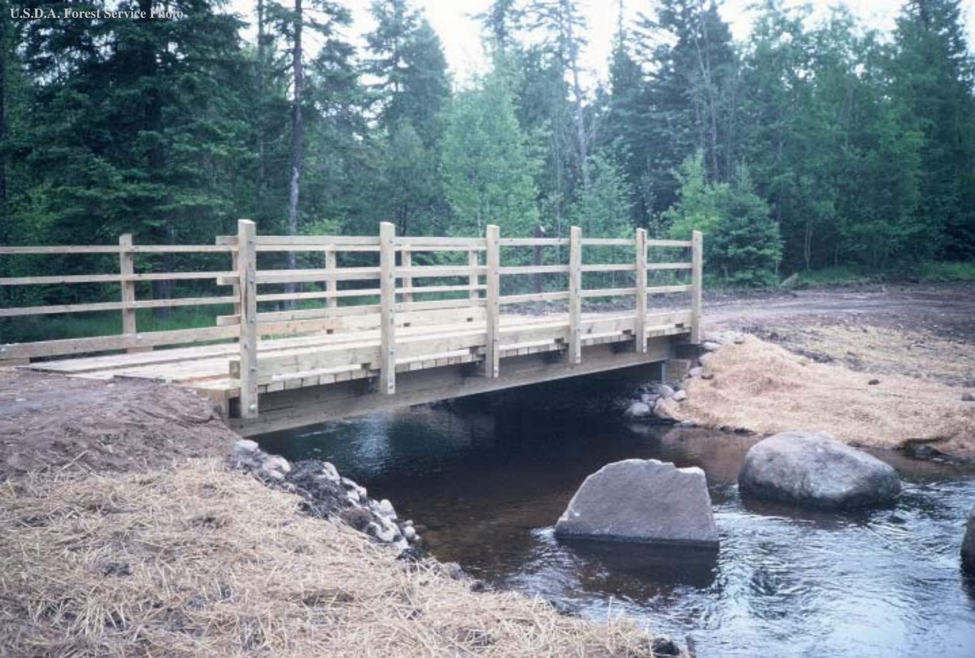
Pipeline North Bridge Completed
