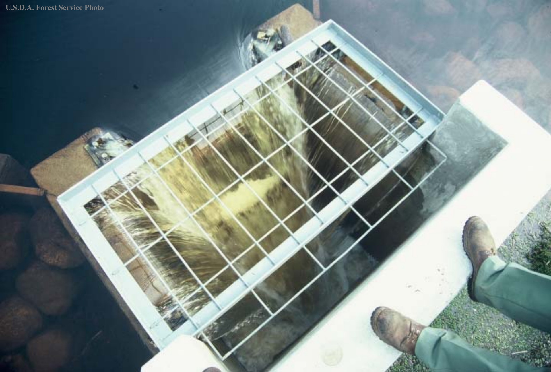
New Water Control Structure, Autumn 1991
