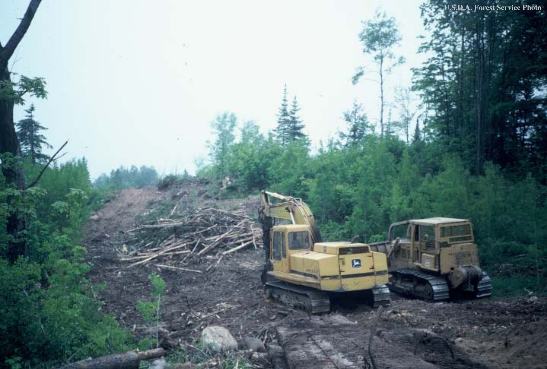
A.N.R. Pipeline Construction Equipment
