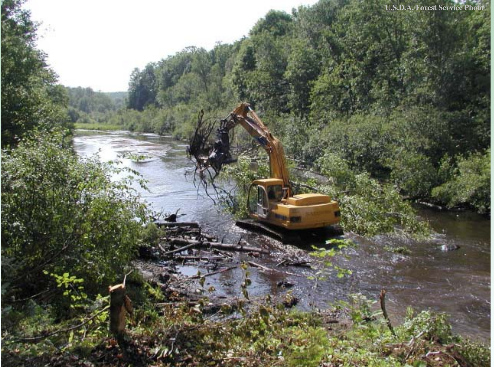
Knowles Dam Removal – Tree in Excavator
