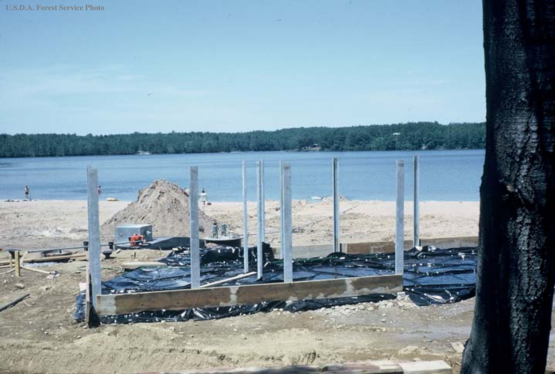
Bass Lake Change House Construction, July 1964
