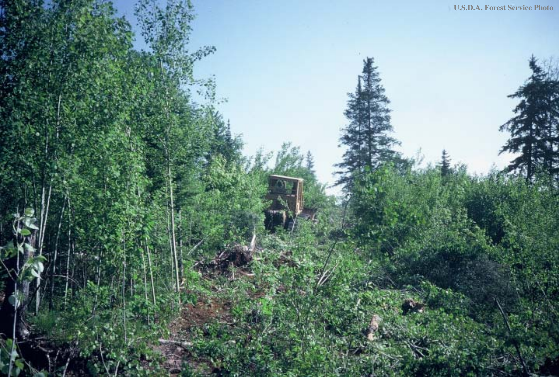
A.N.R. Pipeline Location Before Installation
