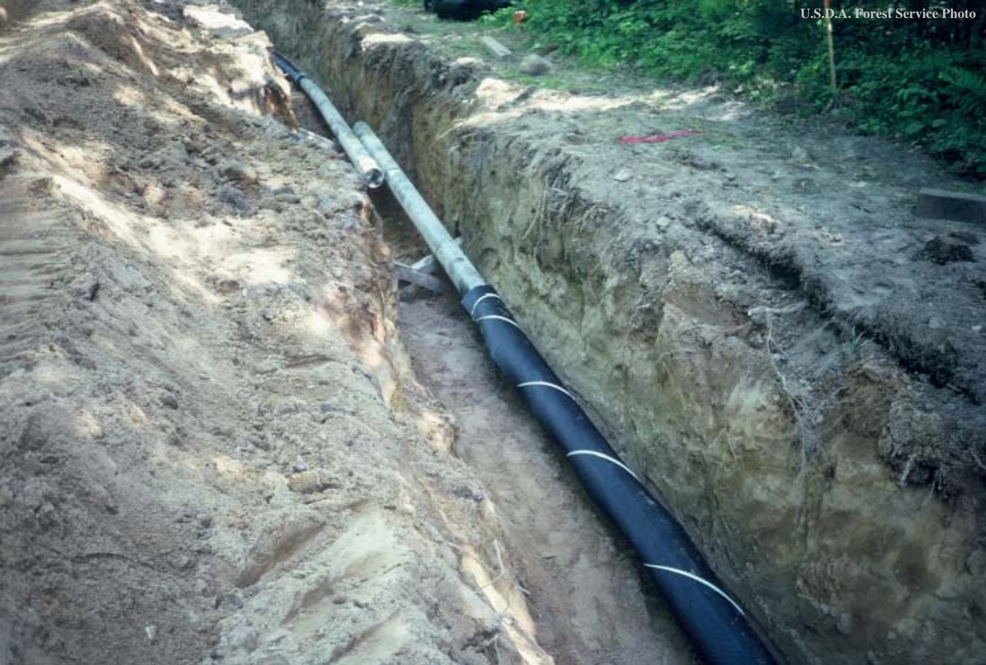
A.N.R. Pipeline - Rock Shield on Pipe
