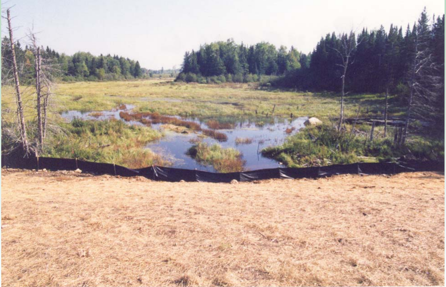
Looking Upstream at Completed Bluegill Creek Impoundment, 1998
