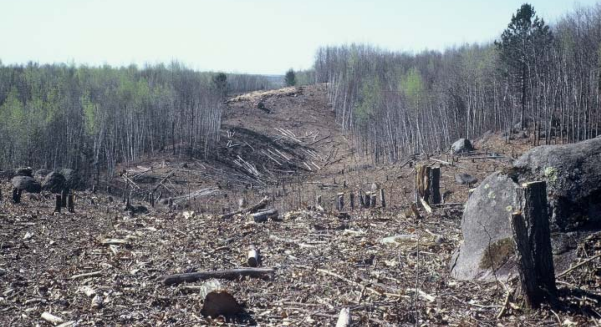
Highway T New Location, May 1964
