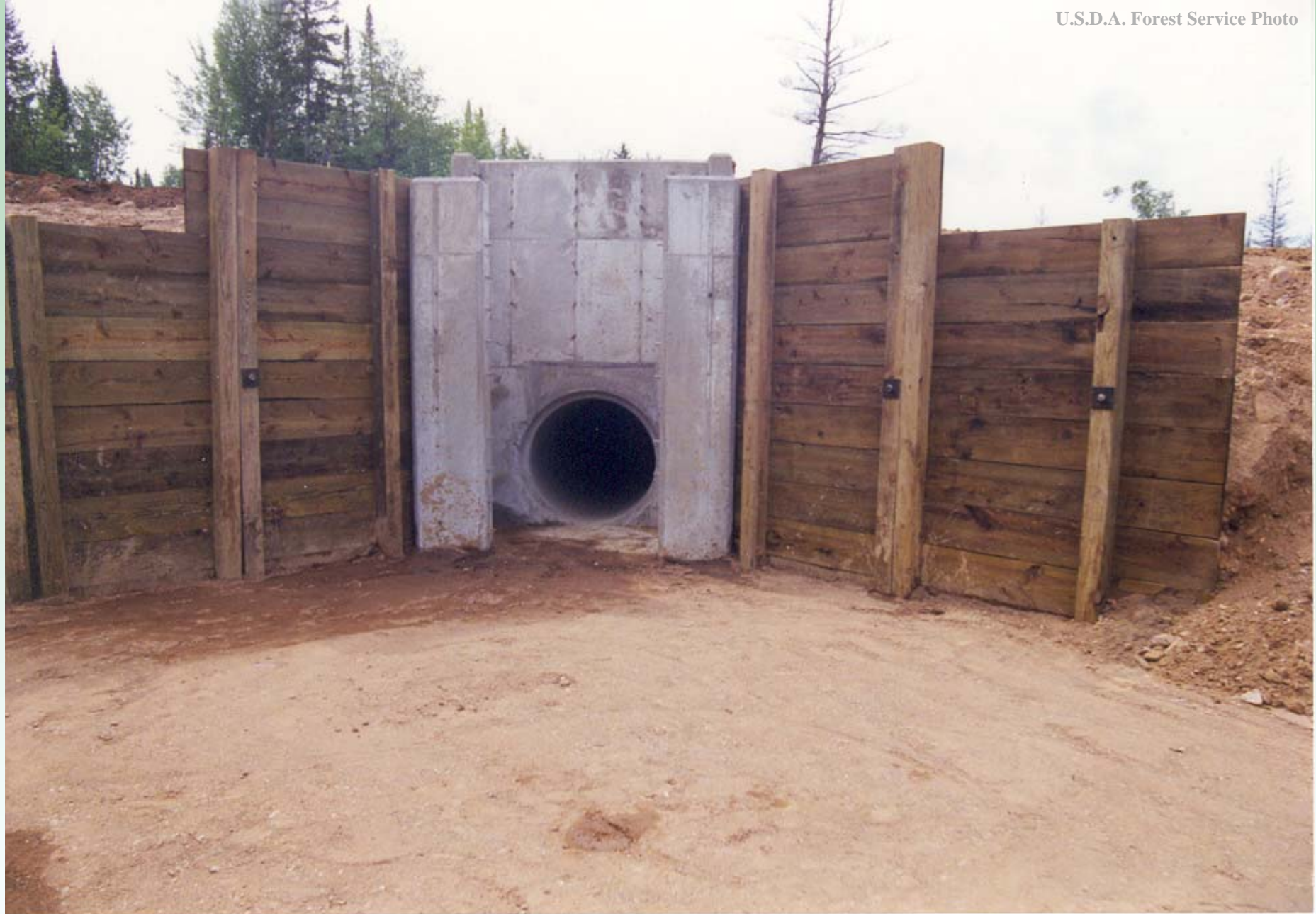
Completed Drop Structure and Wing Walls
