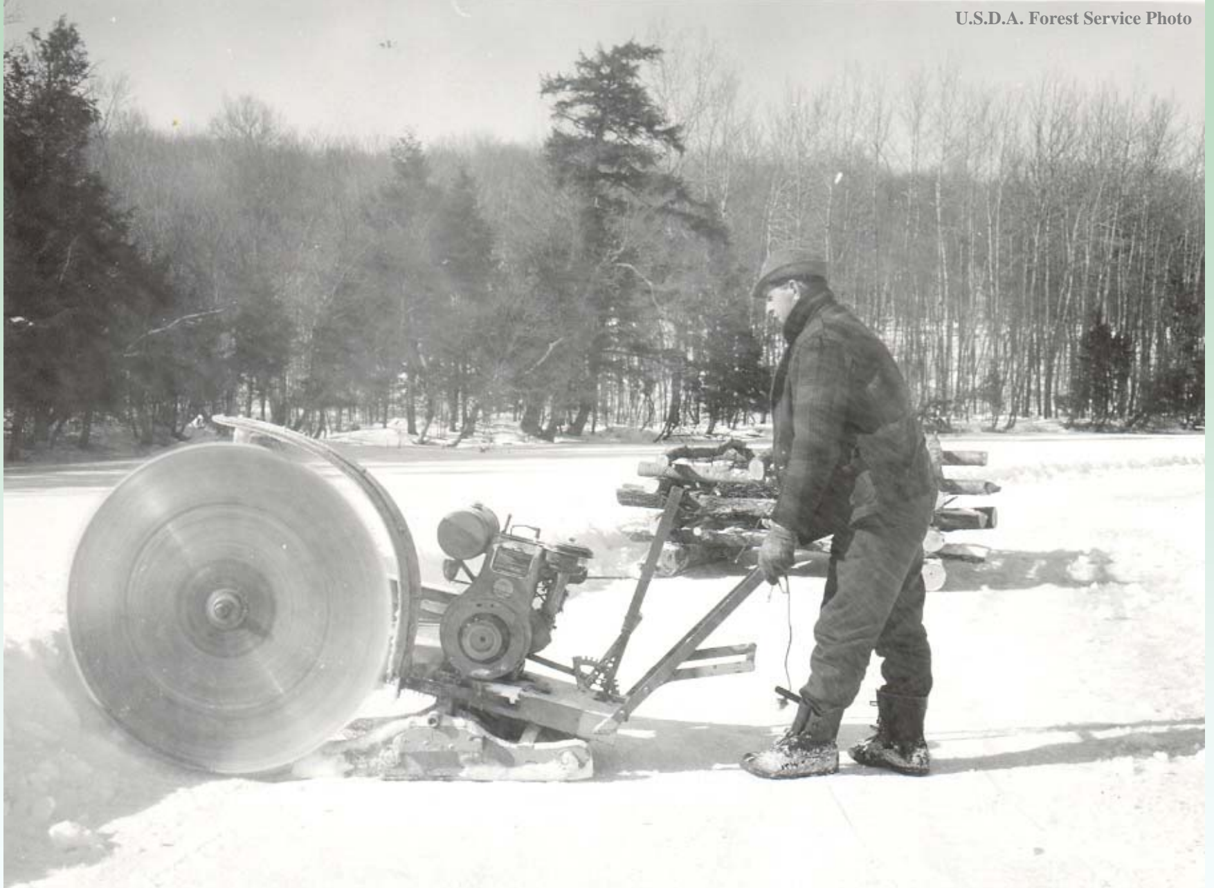
Cutting Ice on Ada Lake for Fish Shelter, February 1963
