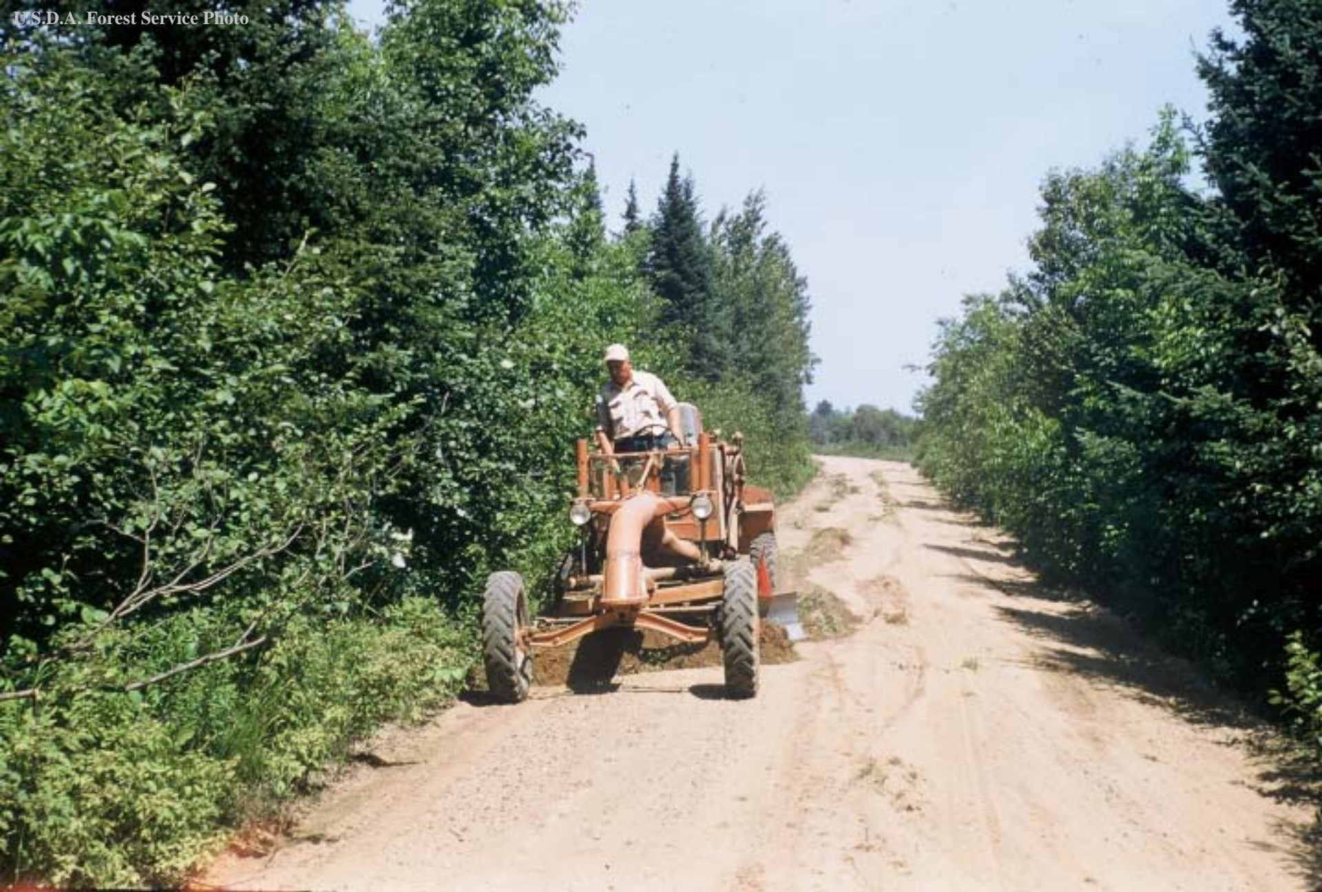
Blading Roads for Maintenance, 1954
