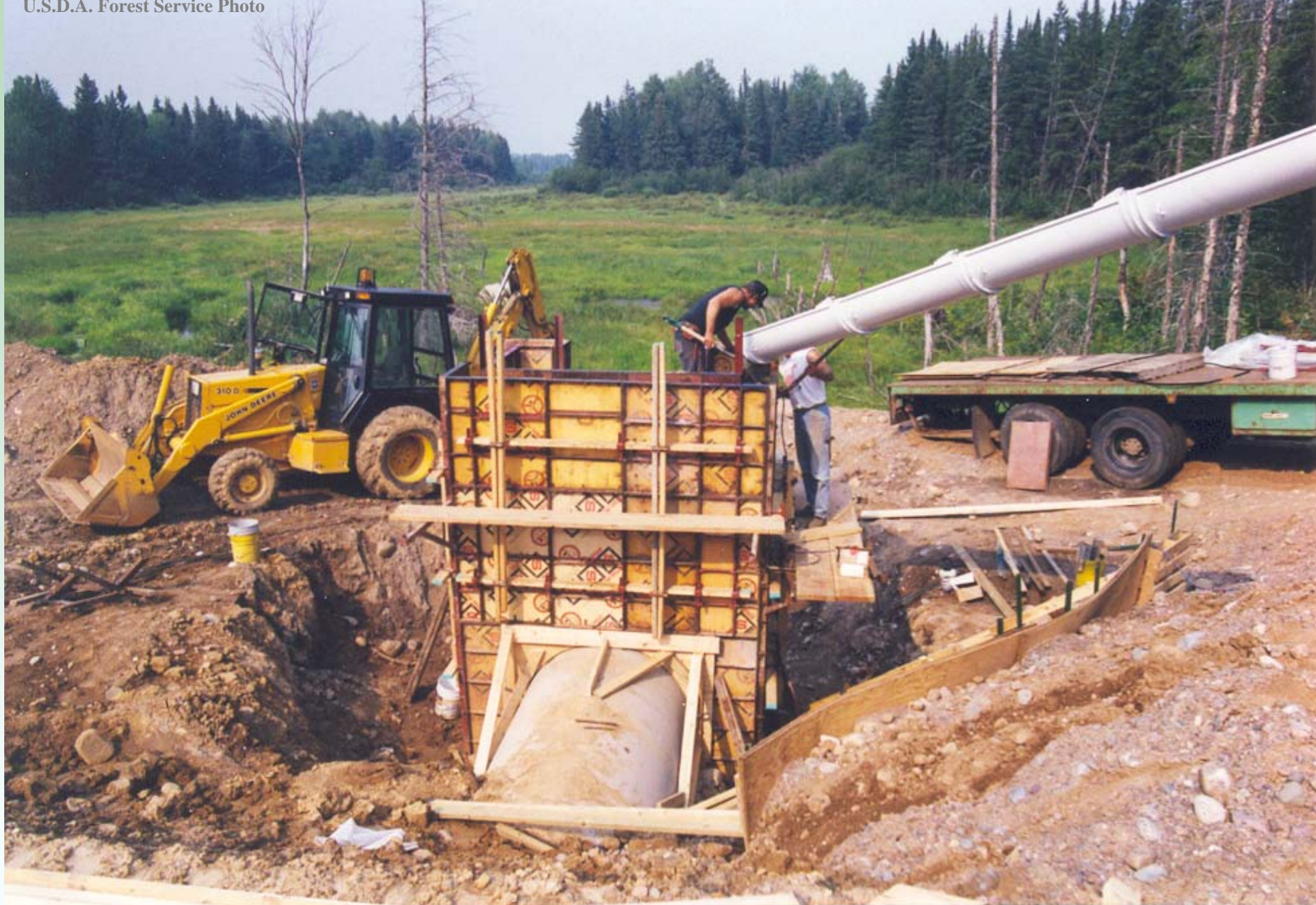
Pouring Concrete to Form Drop Structure
