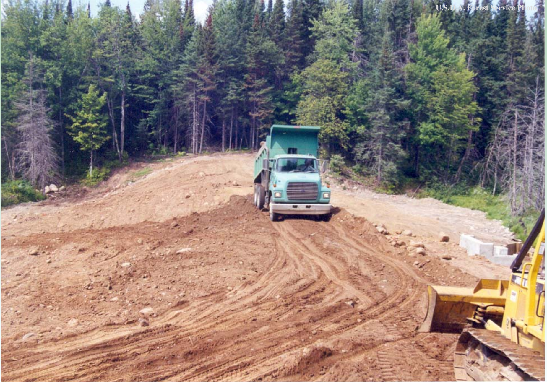
Bluegill Creek Impoundment Construction, 1998
