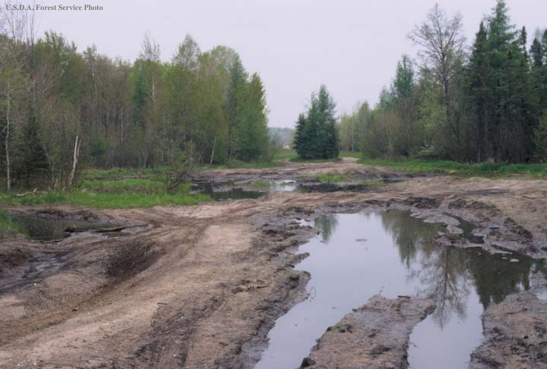
Resource Damage on Pipeline from Recreational Use
