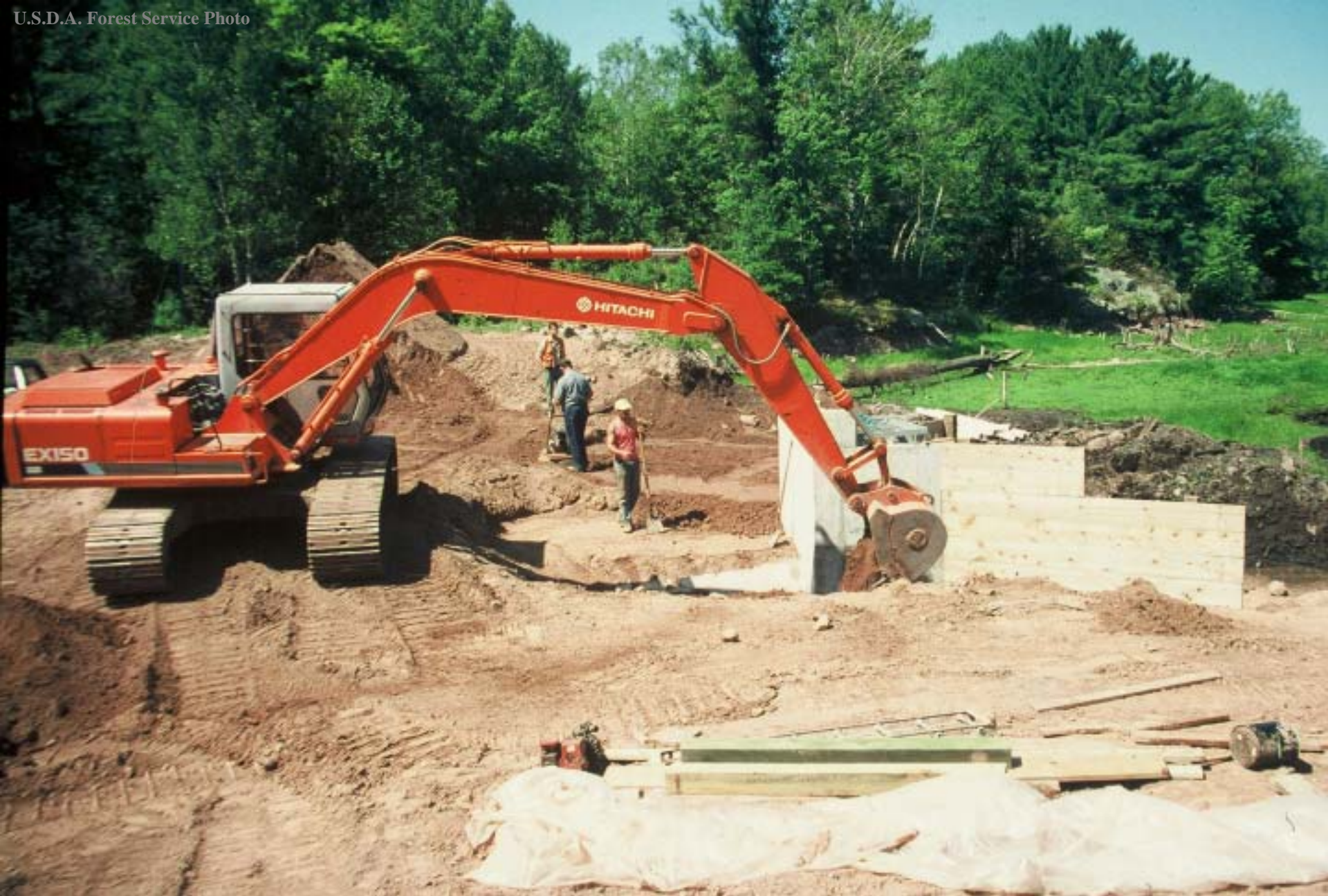
Drop Structure and Wing Walls
