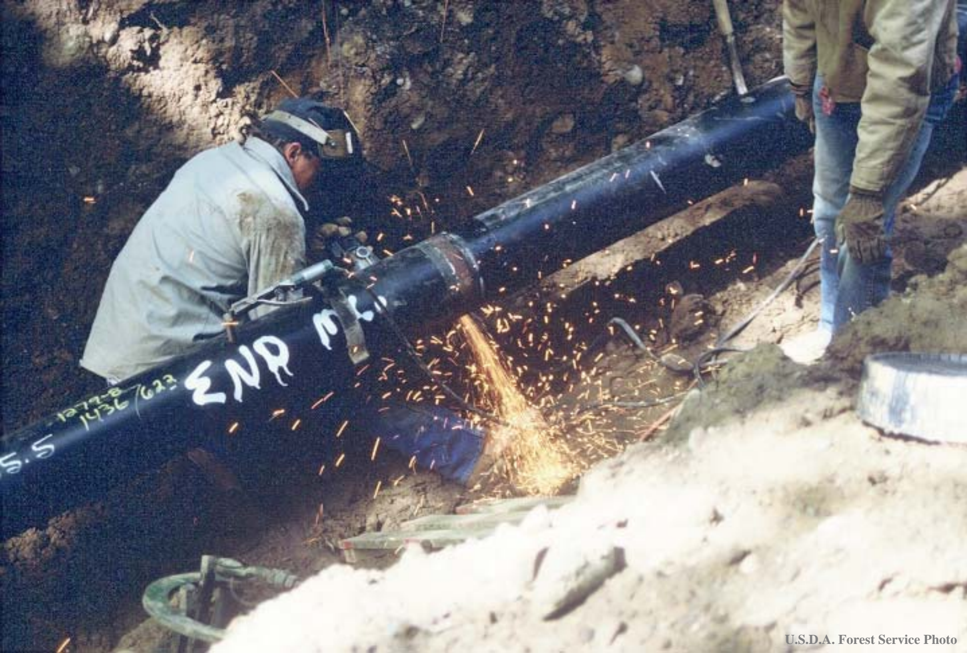
Welding A.N.R. Pipeline
