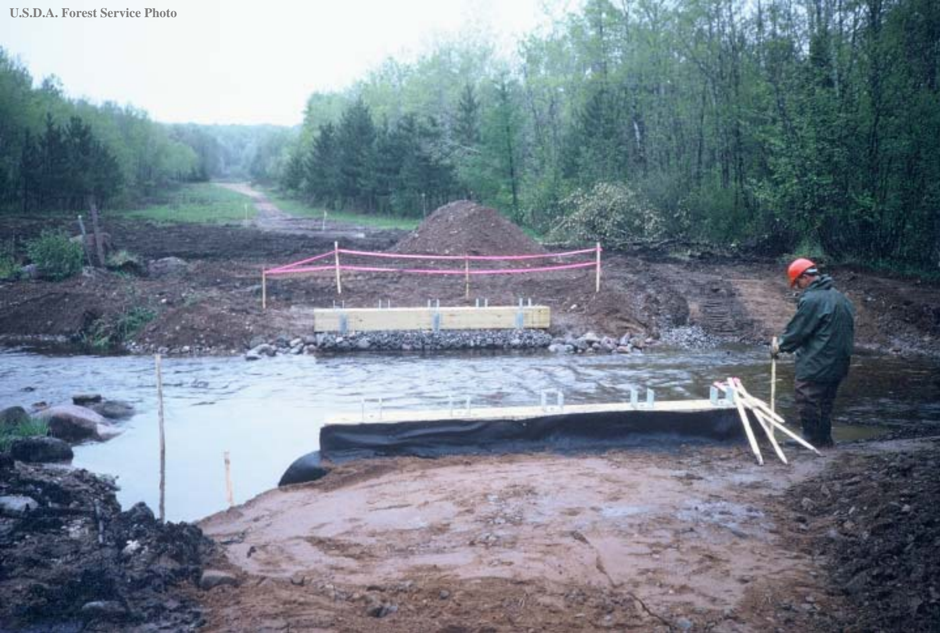
Pipeline Bridge Installation - Abutments on Gabions
