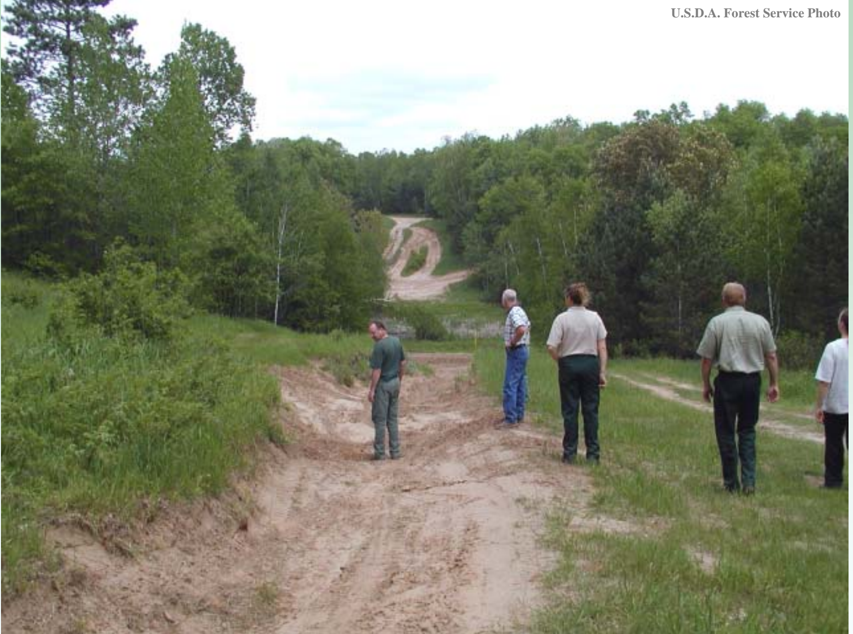
Employees Inspecting Resource Damage on the Pipeline, 2004
