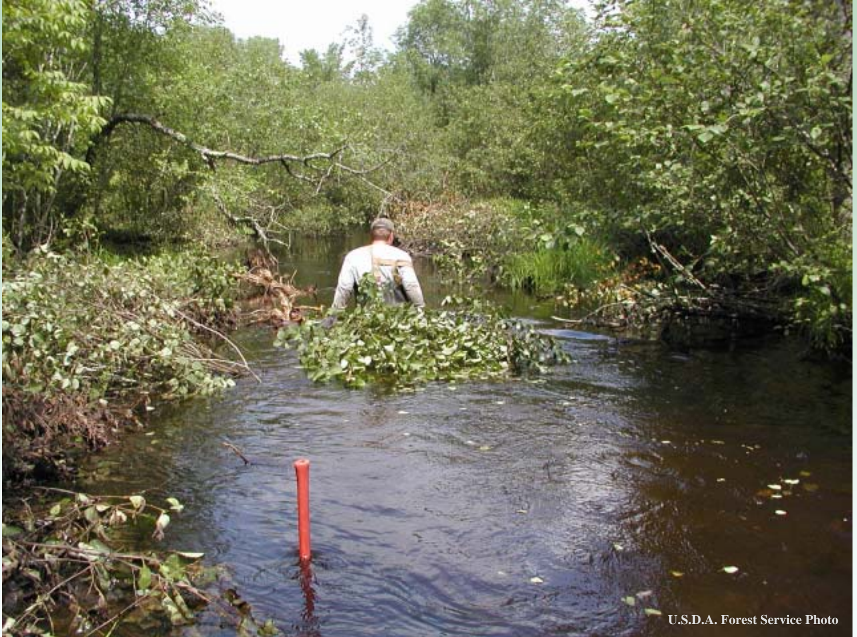
Placing Brush Bundles for Stream Improvement, 2003
