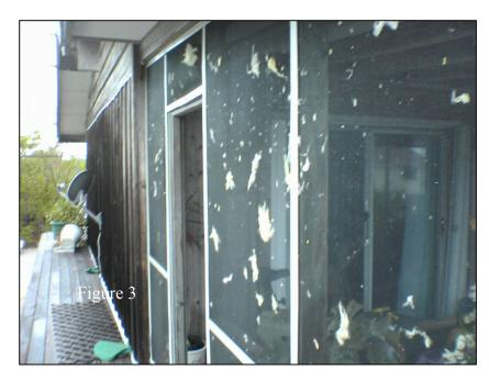
northeast corner of the house where the metal roofing had been peeled away and the underlying framing damaged, and a patio running the length of the back of the house was completely destroyed. Insulation from the roof was found embedded in the screen porch
