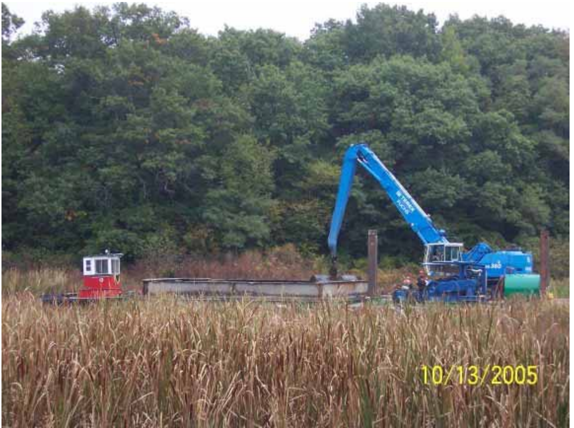
A tug and barge operation removes sediment from the Pond. The majority of contaminated sediment is located in the Pond.
