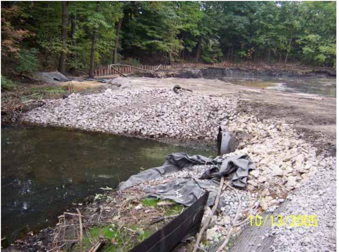
The creek is dammed up and diverted through a culvert.
