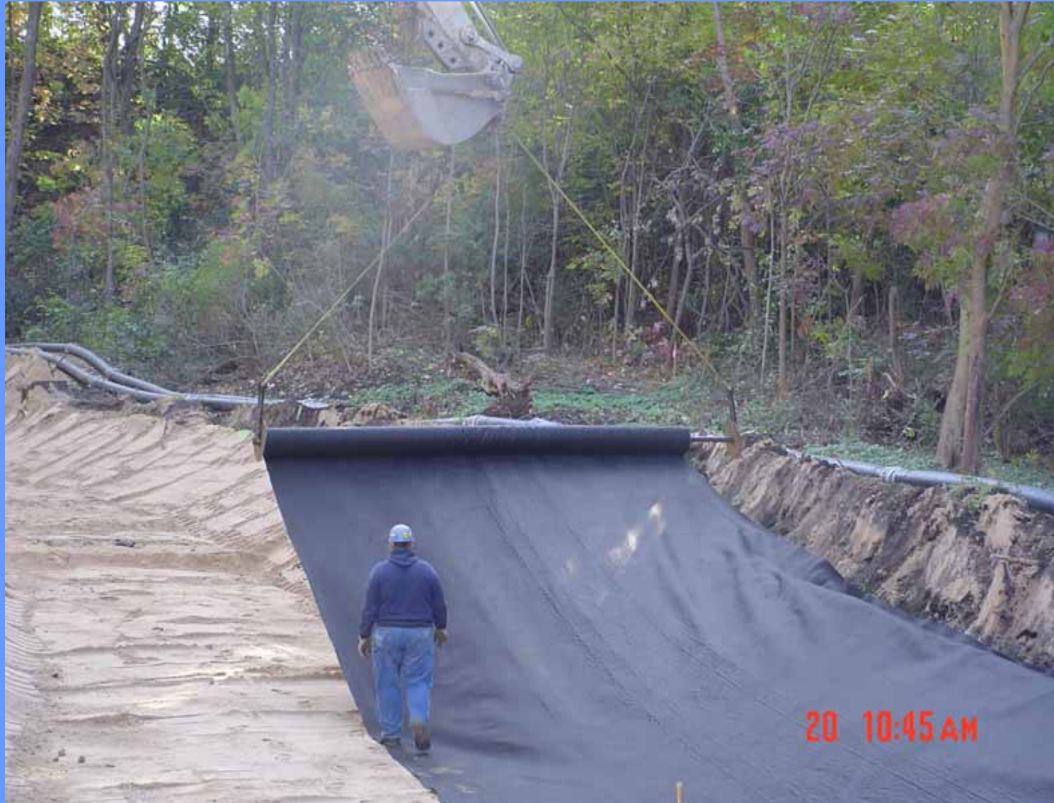
Placing geotextile over sand layer in Ruddiman Creek
