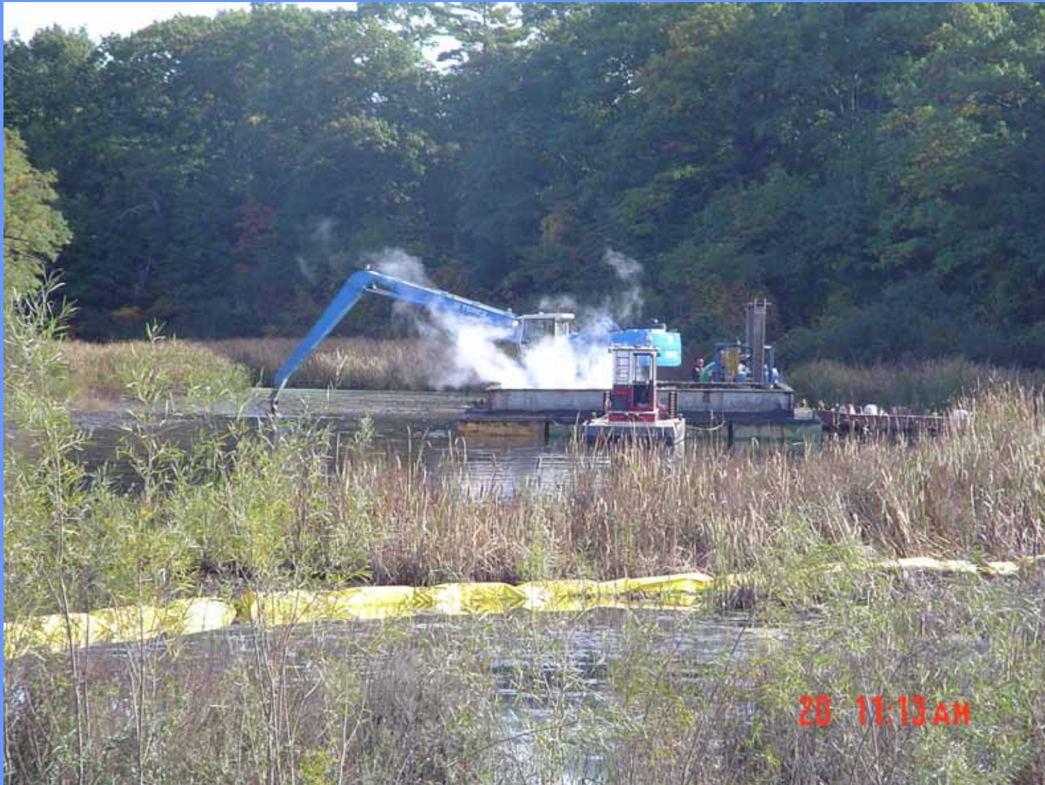
Dredging in Ruddiman Pond
