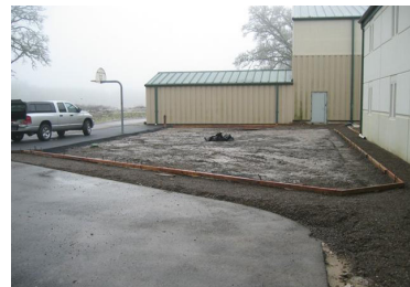
(Above) Construction on the outdoor recreation area continues.
