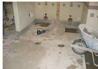
(Above) Demolition work was underway in the bathrooms in preparation for adding privacy screens, new tile flooring, and bathtubs is well underway.
