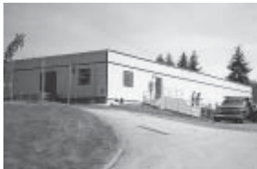
Completed modular facility at Hillcrest.
