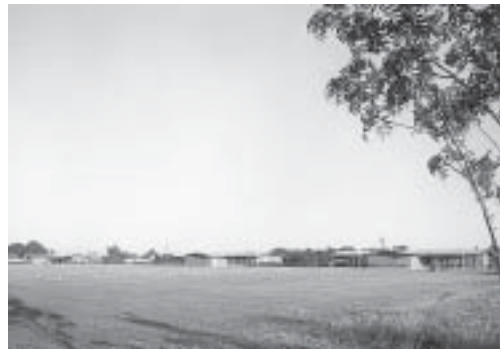
Eight "front cottages" line the drive of the facility grounds. These living/treatment units were constructed between 1960 and 1964.
