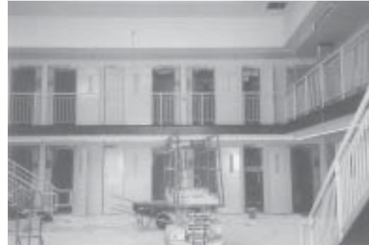
Detention County Housing Unit (Dayroom)
