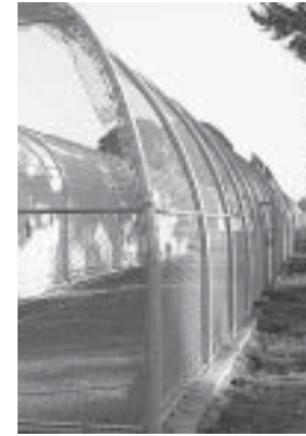
Perimeter of the fenced compound.
