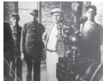
State Reform School's Boiler Room Crew
