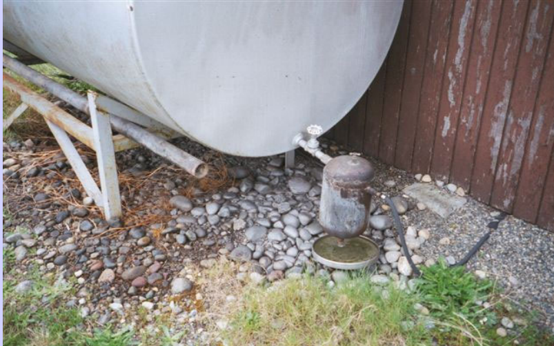
Fuel tank leaking diesel next to wellhead Credit: Rural Community Assistance Corporation
