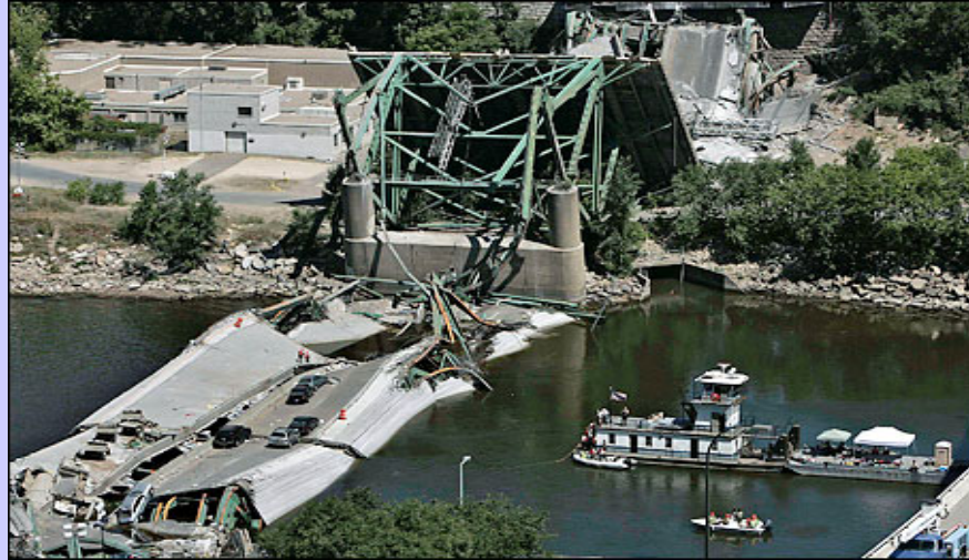
MN bridge collapse, August 2007 Credit: Jim Gehrz, Associated Press
