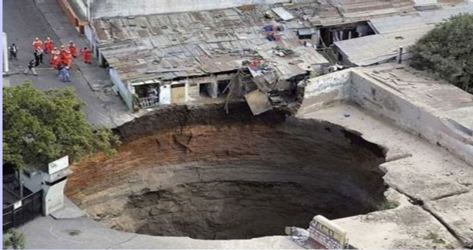
Guatemala Sewer Pipe Explosion, February 2007
