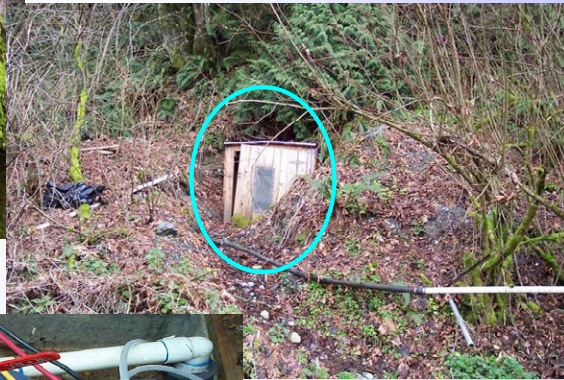
Spring Box with open access
