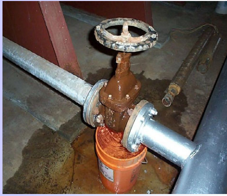
Leaking valve
