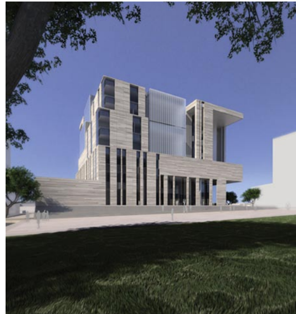
(Future) U.S. Courthouse , Austin, TX
