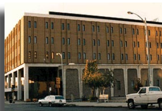
Federal Building and Post Office Fargo, ND
