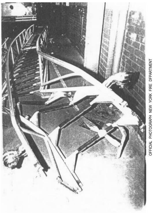
Figure 4. Photograph of the Bed Section of the Failed Ladder Showing the Buckled "Hinges" in the Right Bottom Chord.
