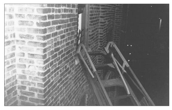
Prior to the collapse, the tip of the left rail rested on the window sill. The weight of the occupants caused a twisting force to the unsupported right side.
