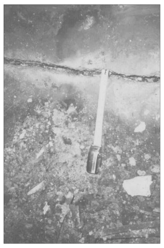
Close-up of crack in concrete floor, 28th floor.
