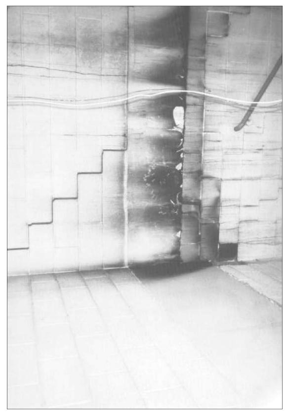
Fire tower between 25th and 26th floors. Note heavy fire and smoke damage.
