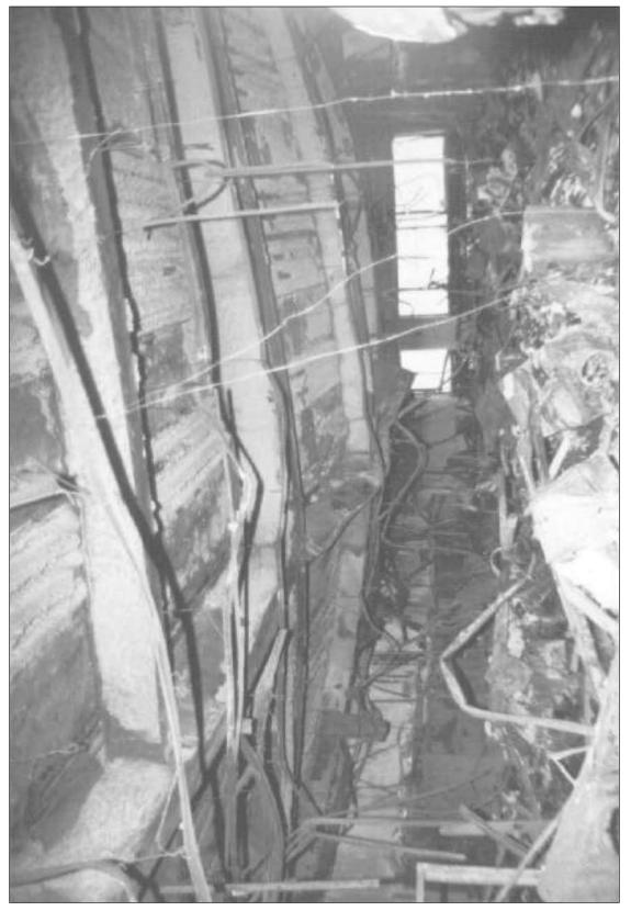
Here and in the next three photos are interior views of floor areas after the fire. Note the total consumption of the available fuel and sagging of the floor deck of up to three feet between columns.
