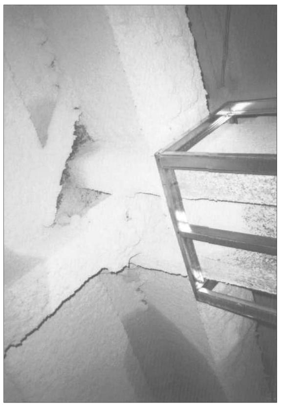
Detail of typical Type 1B construction, 6th floor. Note the spray-applied fireproofing and framing for gypsum wallboard.
