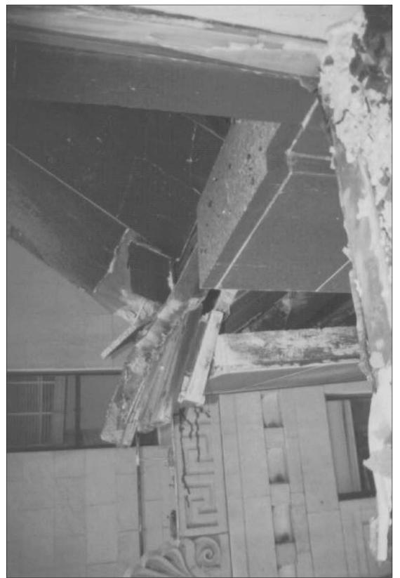
Here and in the next two photos exterior granite panels from the east stair tower were dislodged due to the thermal expansion of the steel frame of the building.
