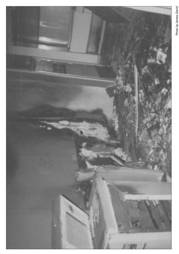
One of the areas of fire penetration on the 30th floor where a single sprinkler head activated to stop the upward extension of the fire.
