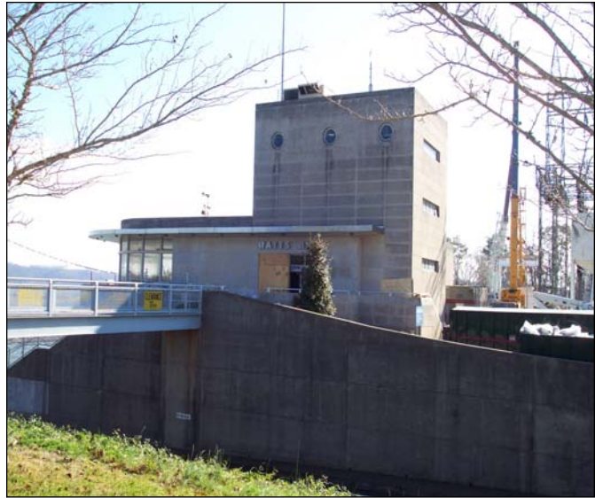
View of the Control Building from across Route 68
