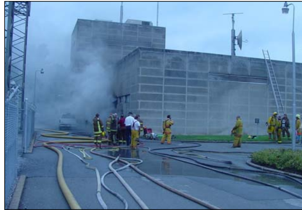
View of the control building from the South. Note the solid concrete construction and lack of windows.
