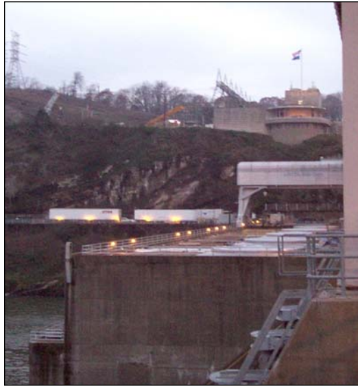
View of the Control Building from the Dam
