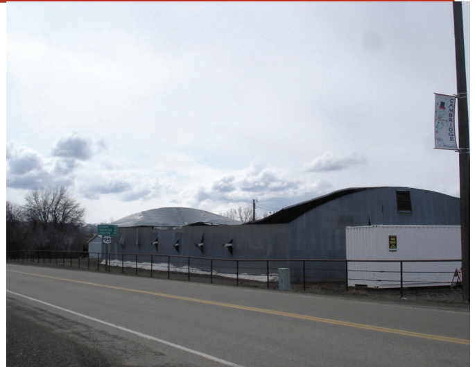
Figure 3. Building crushed by snow in Cambridge, Idaho.
