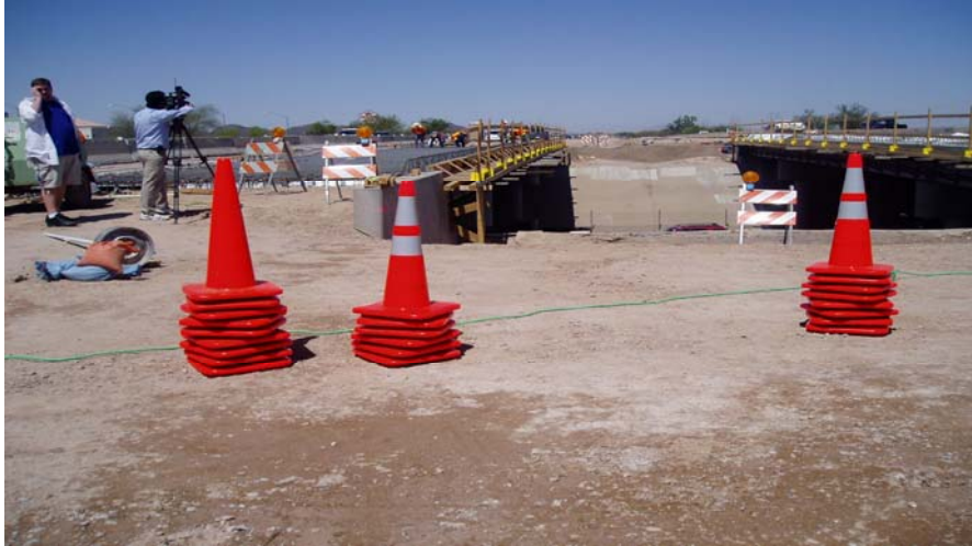
Active Work Zone Site
