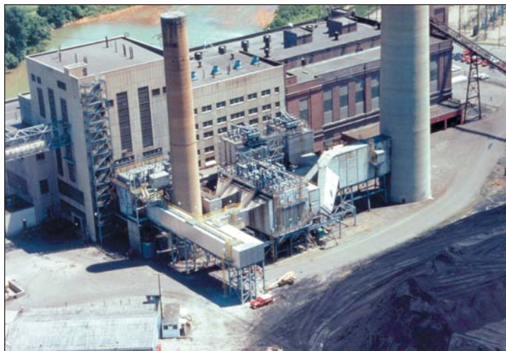
Bechtel's demonstration showed that 50% \text{SO}_2 removal efficiency was possible using CZD/FGD technology. The extended duct into which lime slurry was injected is in the foreground.
