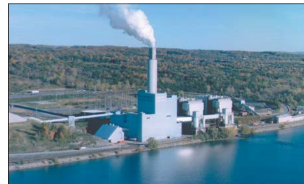
Milliken Station served as the host for two CCTDP projects demonstrating advanced environmental controls.
