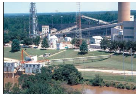
SO 2 control technologies: AirPol (left), CT-121 (center), and LIFAC (right).
