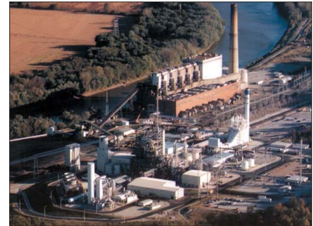
Wabash River Coal Gasification Repowering Project (Wabash River Coal Gasification Repowering Project Joint Venture)—1996 Powerplant Award presented by Power magazine.
