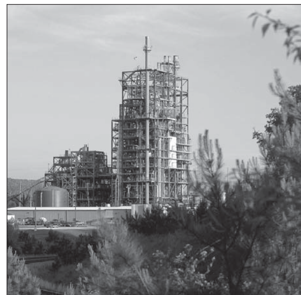
The PSDF facility in Wilsonville, Alabama.
