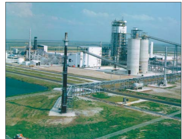
Tampa Electric Integrated Gasification Combined-Cycle Project (Tampa Electric Company)—1997 Powerplant Award presented by Power magazine.
