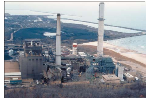
Advanced Flue Gas Desulfurization Demonstration Project (Pure Air on the Lake, L.P.)—1993 Powerplant Award presented by Power magazine.
