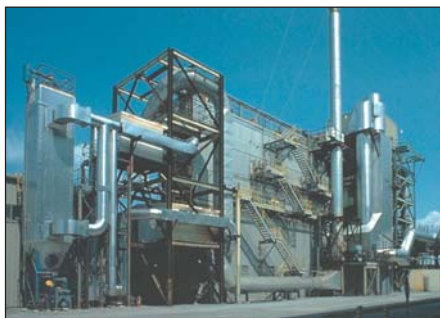
SO 2 control technologies: AirPol (left), CT-121 (center), and LIFAC (right).
