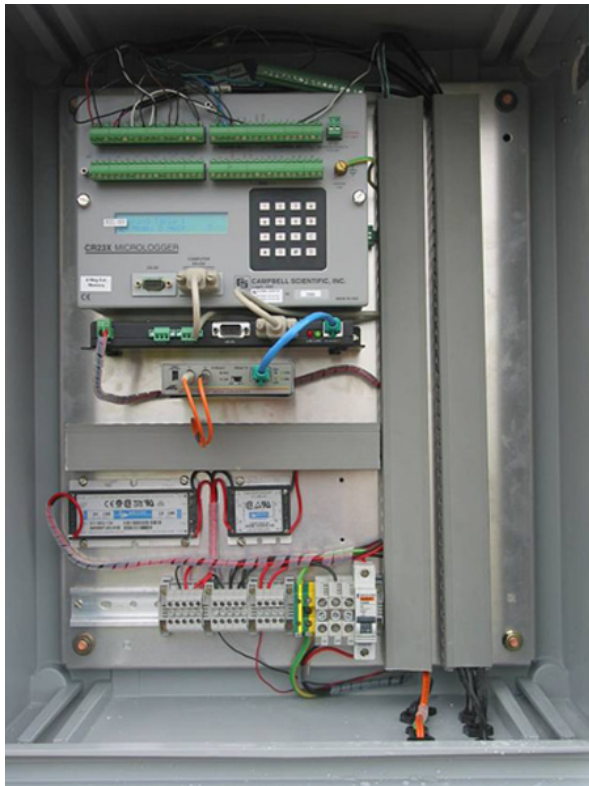
Figure 3. Field installation of the Campbell Scientific, Inc., CR23X data logger and peripherals for the GNDRAD system at Darwin Australia TWP site (left). Removable connectors on the CR23X data logger make for simplified logger change outs (right).
