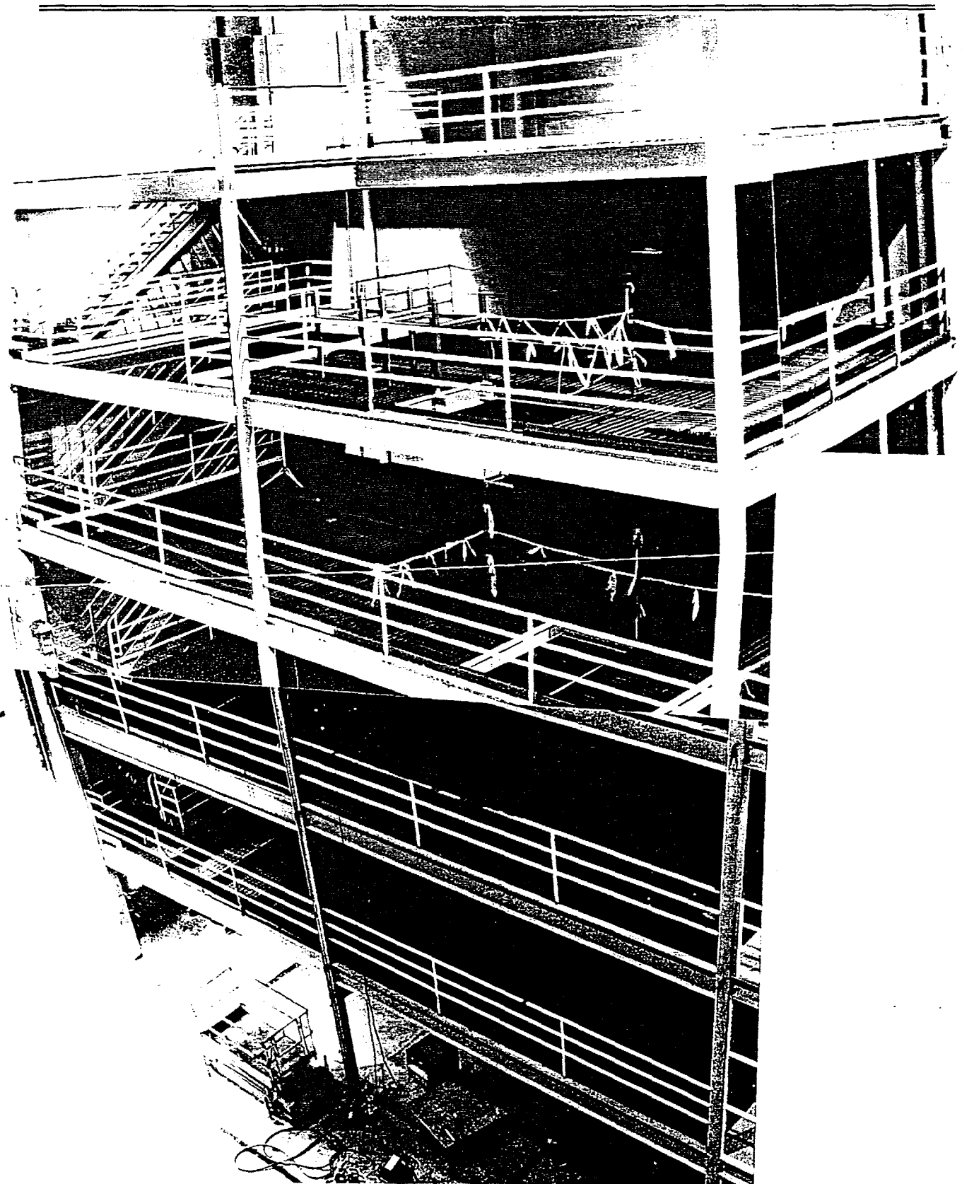
Photograph Illustrating the Progress of the Structural Steel Exhibit 2.2-6
