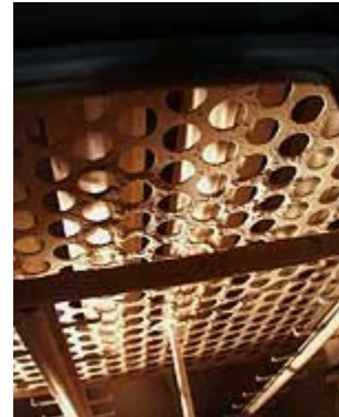
Internal view of the Advanced Hybrid Particulate Collector showing the Gore fabric filter bags, electrodes, and collecting plates.
