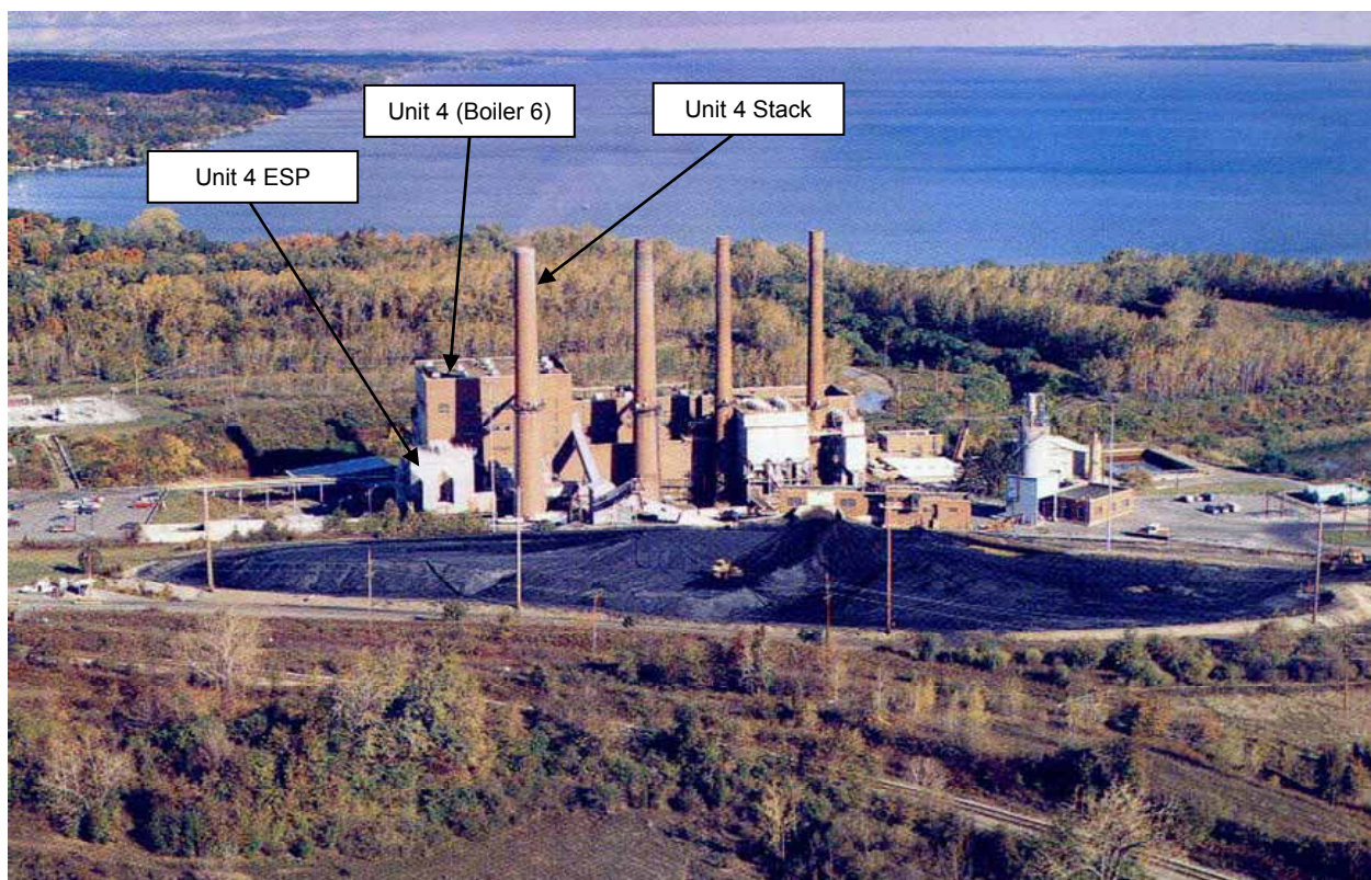
Figure 2. Aerial photograph of the AES Greenidge plant, as viewed from the south.
