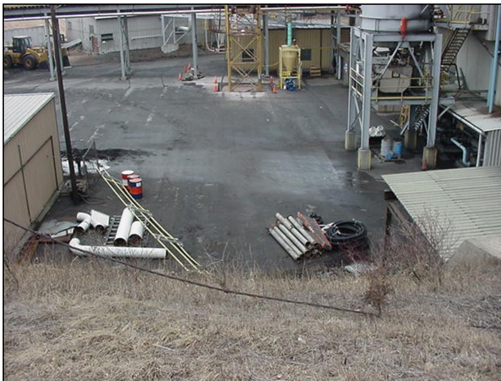
Figure 2.1.4. Photograph of the site for the proposed project at Greenidge Station, as viewed toward the northwest.
