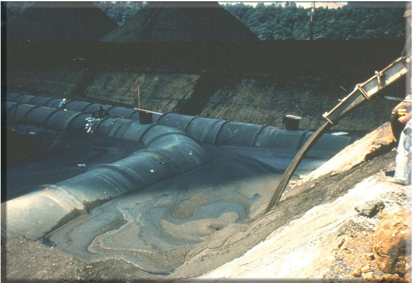
Flowable fill typically contains fly ash and water and may contain small amounts of Portland cement.
