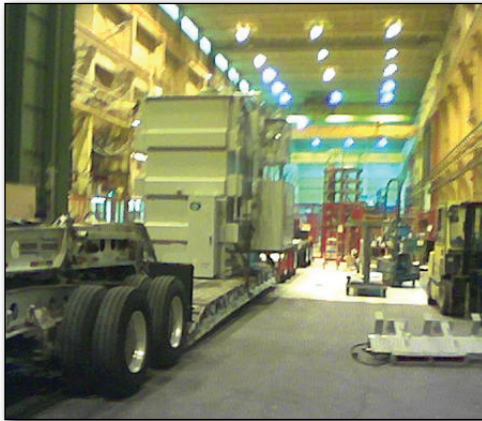
Mobile transformers must be compact enough to fit on a semi-trailer.
