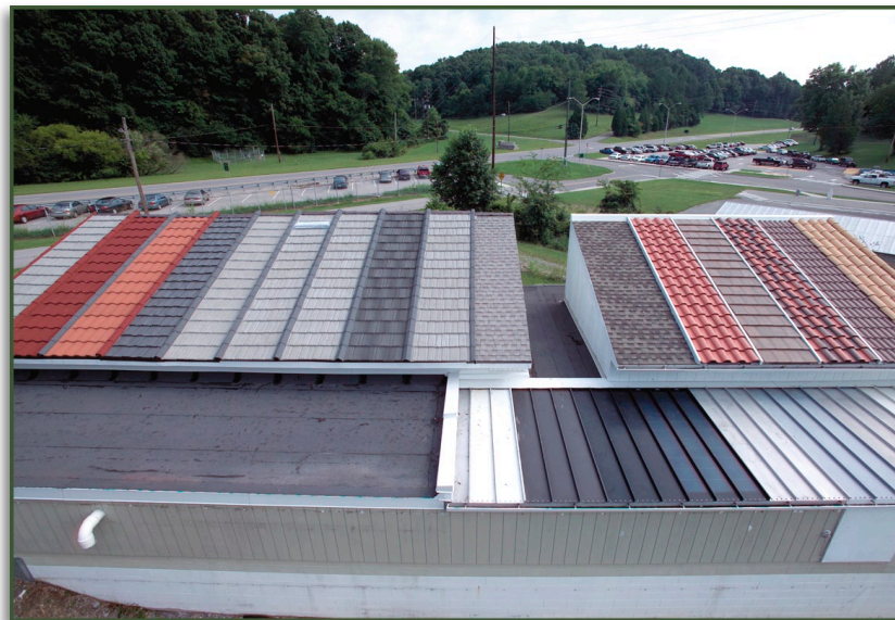
South-facing steep-slope attic assemblies placed atop the roof-testing facility.
