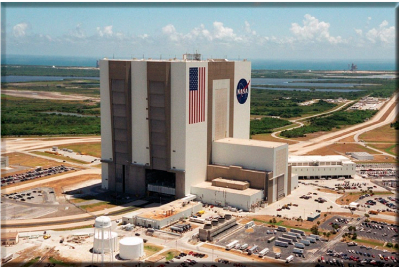
More energy-efficient boilers are projected to save $800,000+ yearly at Kennedy Space Center.
