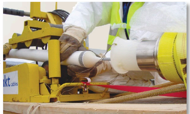
Pulling the HTS cable into the cryostat.
