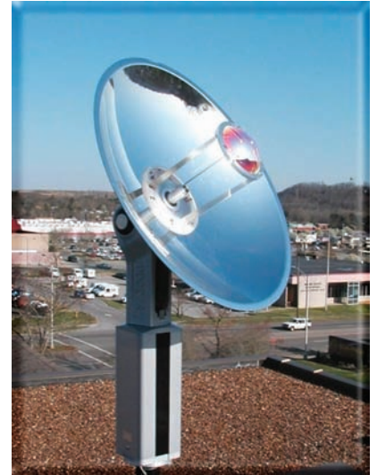
Solar tracker installed at the American Museum of Science and Energy.
