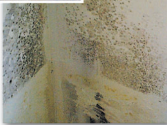
Flooded module (above) and drywall with mold and mildew growth after being under water.
