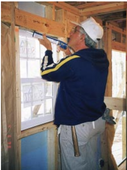
A Habitat volunteer caulks around a window to reduce air leakage.
