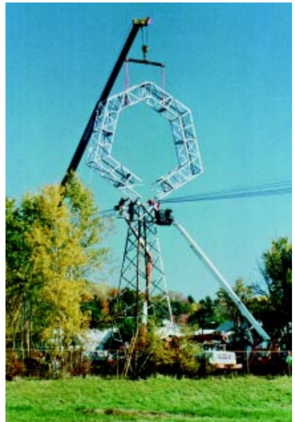
Compact configuration for high phase order lines.
