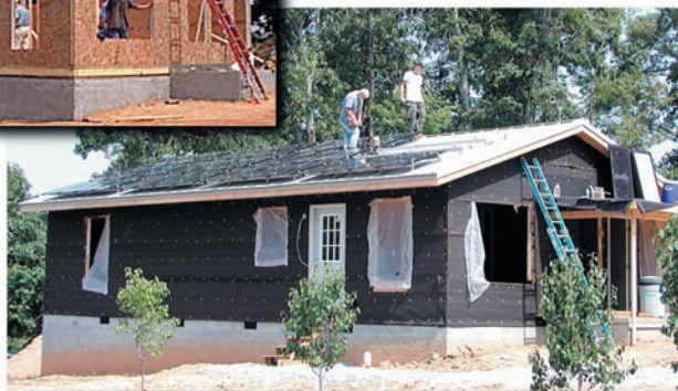
(Right) Solar panels on the roof will generate electrical power for the home. Any surplus power can be sold to TVA.
