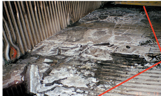
Schematic of recovery boiler floor showing location of cracking in tubes and panels (top) and boiler floor showing the residual smelt bed present during a shut down (bottom).
