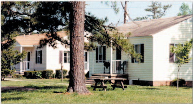
GHP retrofits for military family housing like this account for much of the federal investment in GHPs, more than $200 million to date.
