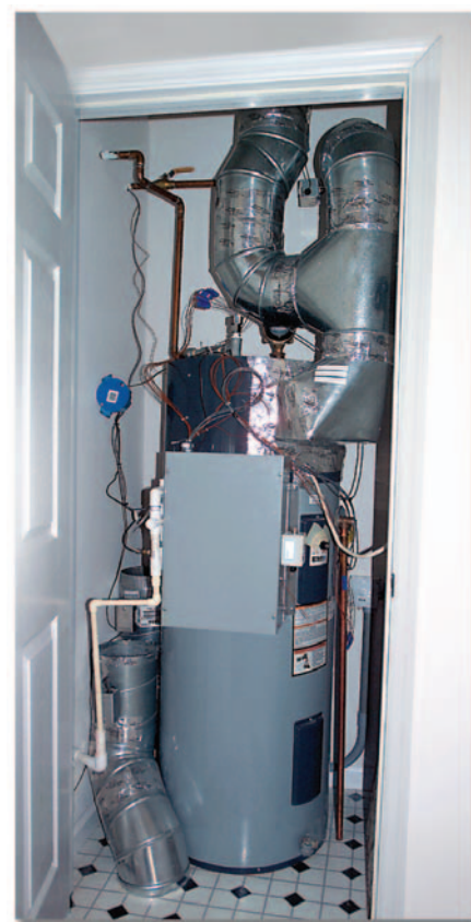
The heat pump water heater uses waste heat from other appliances to preheat water.
