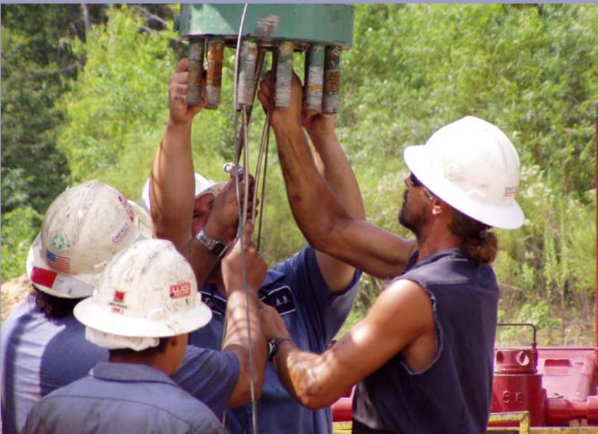
Workers Thread Monitoring Lines Through An Injection Well-Head at the Frio Site (Photo: SD Horvorka, BEG USG UT)
