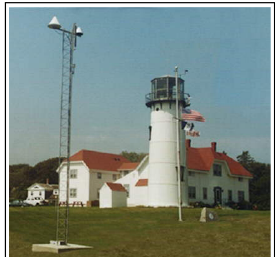
GPS Continuously Operating Reference Station (CORS) located near the Chatham Lighthouse, Massachusetts. This CORS station is one of 650 stations in the national CORS network managed by NOAA in cooperation with numerous partners. NOAA makes data from CORS publicly available to provide users with 3-dimensional positioning with an accuracy of a few centimeters.
