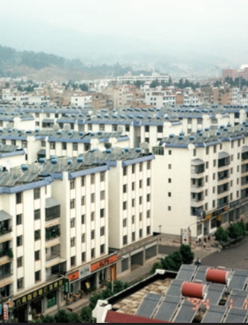
Solar water heater systems on rooftops in Kunming, Yunnan Province, China.
