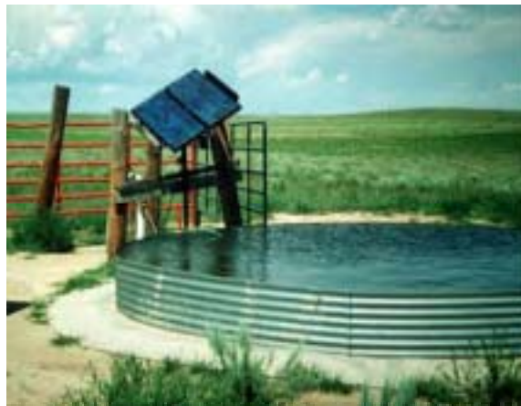
Figure 2-1. PV-powered water pumping on a Colorado Ranch
