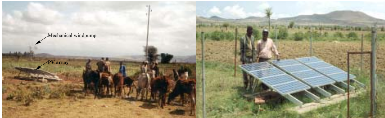
Figure 5-5. An irrigation PV pump in Ethiopia. The pump is also used for livestock watering while the system is not in use.
