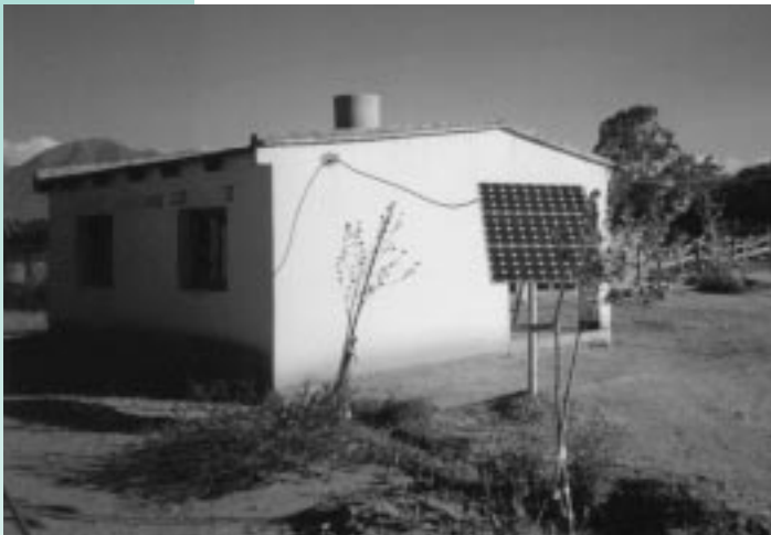
Figure 6.4. A PV system provides electricity to this rural school in Salta province, Argentina.
