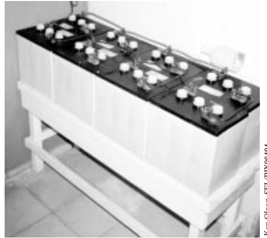
Figure 3.9. Batteries allow an RE system to provide 24 hour power. Photovoltaic panels or a wind generator can recharge the batteries.
