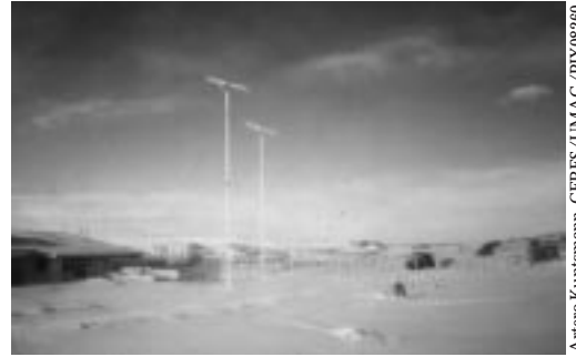
Figure 6.5. Two 1.0 kW wind turbines provide electricity to the dormitory of this remote school at Villa Tehuelche.
