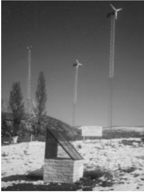
Figure 3.5. Small wind turbines, solar oven, and radio tower at the Las Cortaderas Primary School 250 km west of Neuquén, Argentina.
