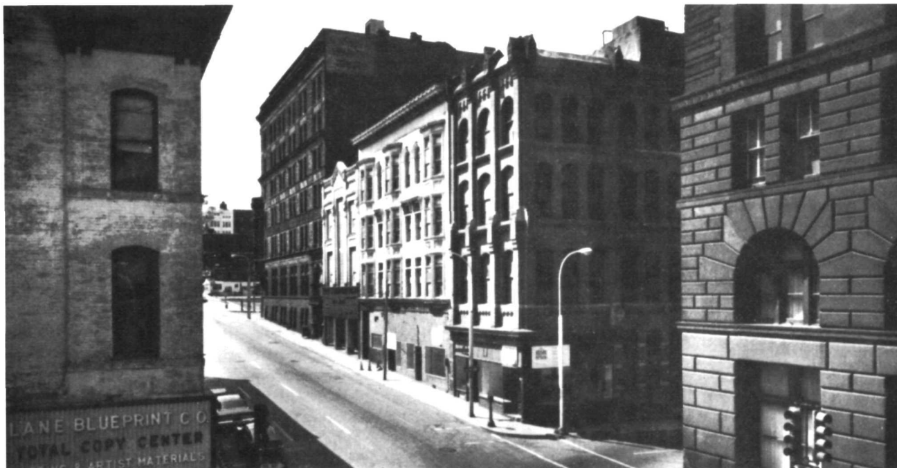
Older commercial buildings in downtown areas are particularly vulnerable to decay and demolition yet could be successfully rehabilitated. This downtown block, in Kansas City, Missouri, is listed in the National Register of Historic Places as part of the West Ninth Street/Baltimore Avenue Historic District. (Paul S. Kivett)
