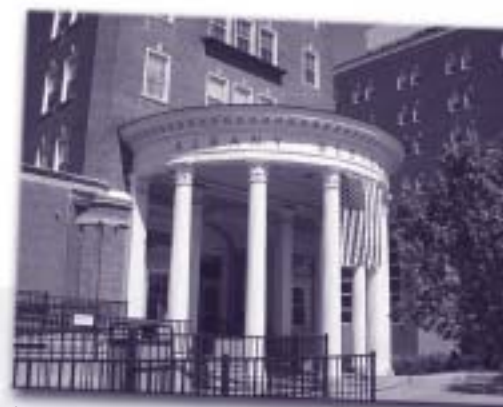
The Albany Medical Center has reaped energy savings for 10 years.
