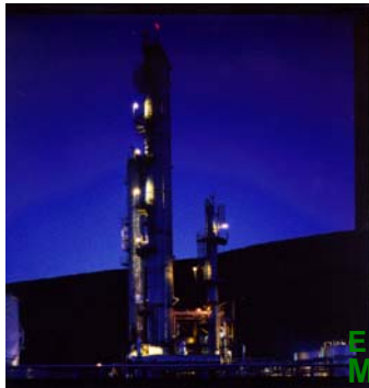
Kingston, Jamaica Ethanol Plant
