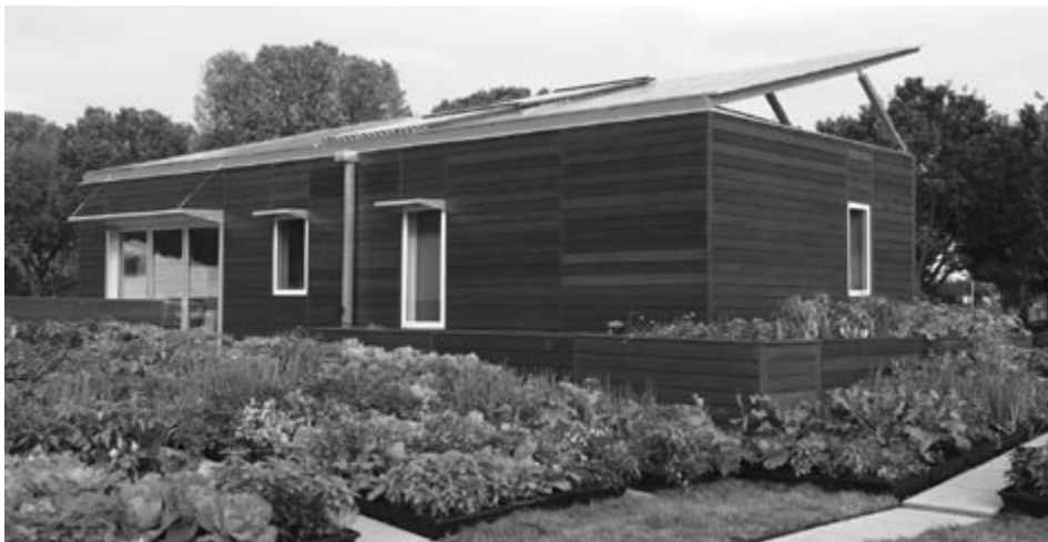
The Architecture jury praised the Cornell University house, commenting that the crisp building set in a lush edible landscape made a great initial impression.
