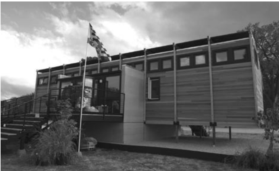
The Maryland house was the “People’s Choice Award” winner of the 2005 Solar Decathlon. The Dwelling contest judges commented that the house feels big and comfortable, with a kitchen layout that is very usable.
