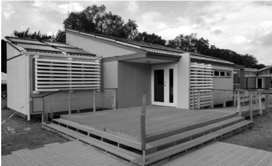
The Puerto Rico house has large south-facing windows to maximize the daylight and minimize use of electric lights. Fixed louvers over the windows block radiation, but let in sunlight.
