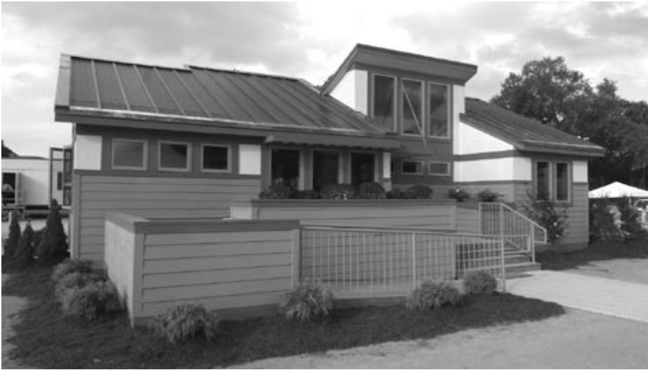
The Missouri-Rolla house design is traditional in its reflection of the work of Frank Lloyd Wright. But it's forward-looking as the only house in the competition that uses thin-film PV panels as the primary power source.
