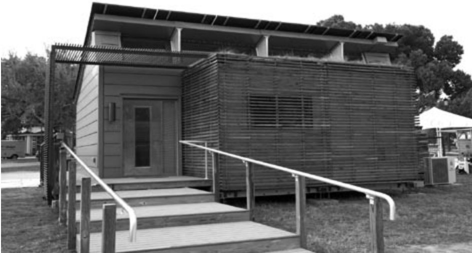
The Texas house consists of prefabricated modules that snap together. The Architecture jury was impressed with the team’s grasp of getting the passive elements right first, before adding high-tech elements.
