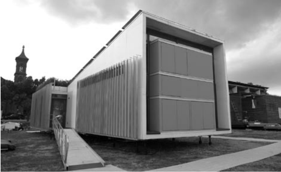
The RISD house is designed for an urban setting and to allow use as a row house. Heliotropic vertical louvers track the sun to keep out unwanted heat.
