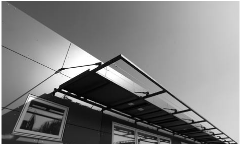
Cal Poly's building-integrated PV awning does double duty as a power source and an attractive design element.
