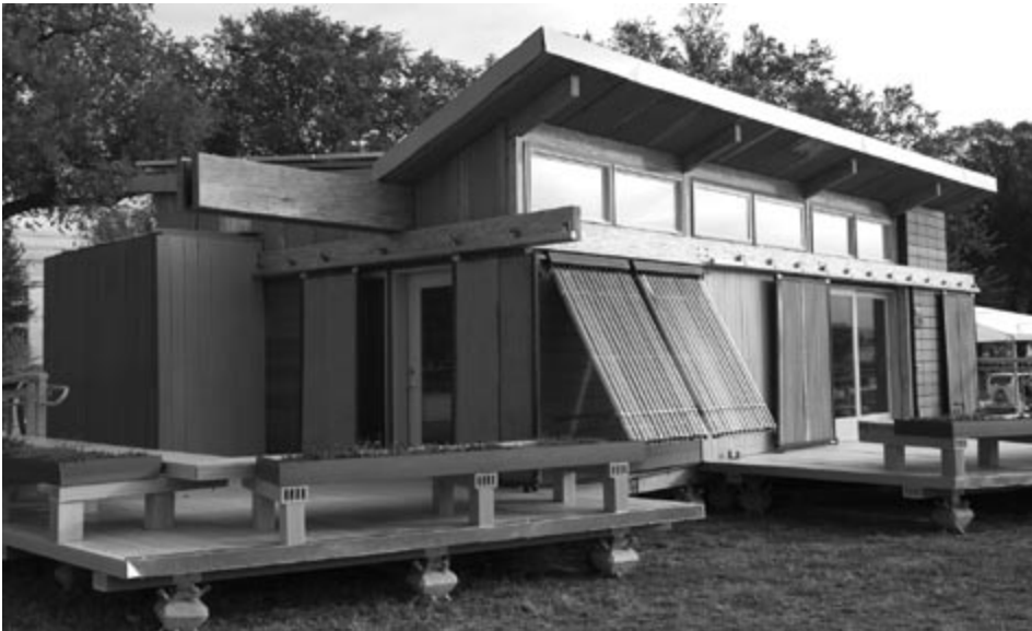
The shipping container in which the Washington State house traveled formed the core of the house on site at the National Mall. The Architecture jury admired the team's exuberance of ideas and the risks taken in their execution.
