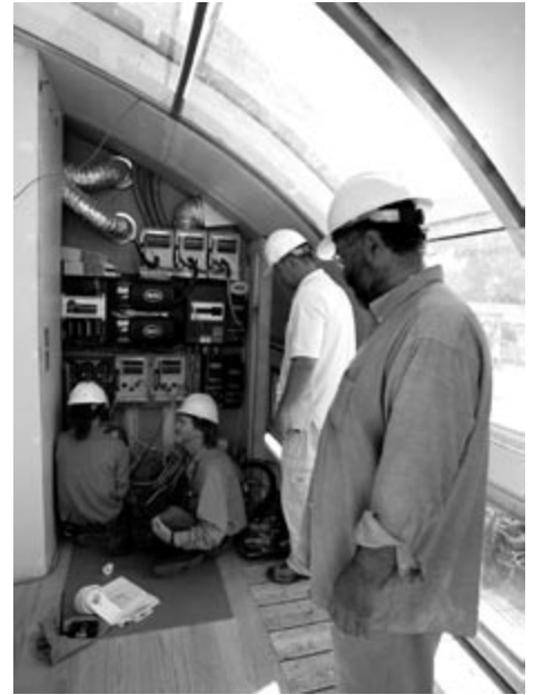
While the students assembled their houses, a team from the National Renewable Energy Laboratory installed monitoring systems to capture data essential to conducting several of the contests. The University of Michigan house is pictured.
