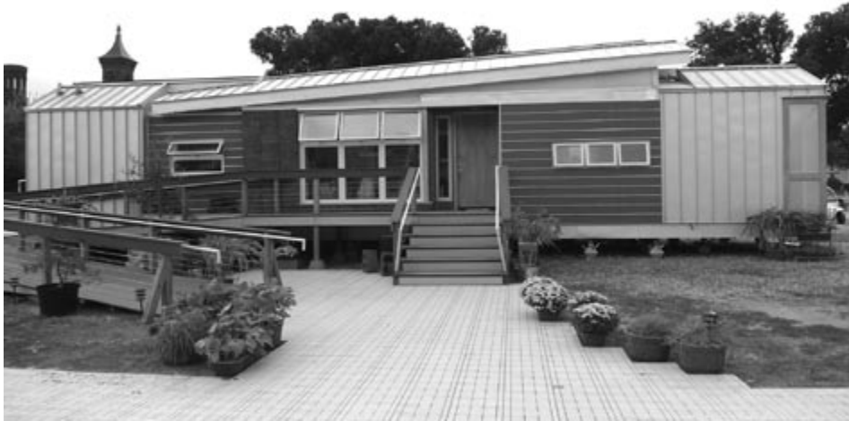
Colorado's home features a movable roof constructed of custom steel struts that lowers for ease of travel and lifts for a feeling of openness and increased lighting when the house is stationary.
