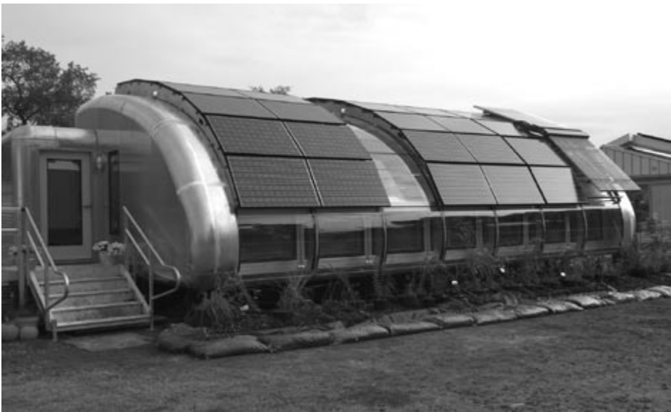
The Michigan house is based on monocoque designs from the aircraft and automobile industries, in which the external skins of an object support some or most of the load of the structure.
