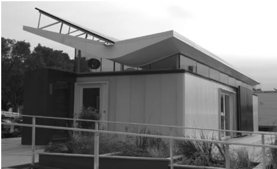
The Virginia Tech home is all about light, from its floating roof, which gestures toward the sun, down through its three translucent walls.
