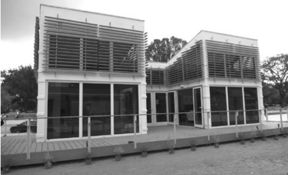
Reflecting Florida's architectural roots, the northern facade of the Florida Intl house is virtually all windows, which are protected by operable louvered blinds to control daylighting.
