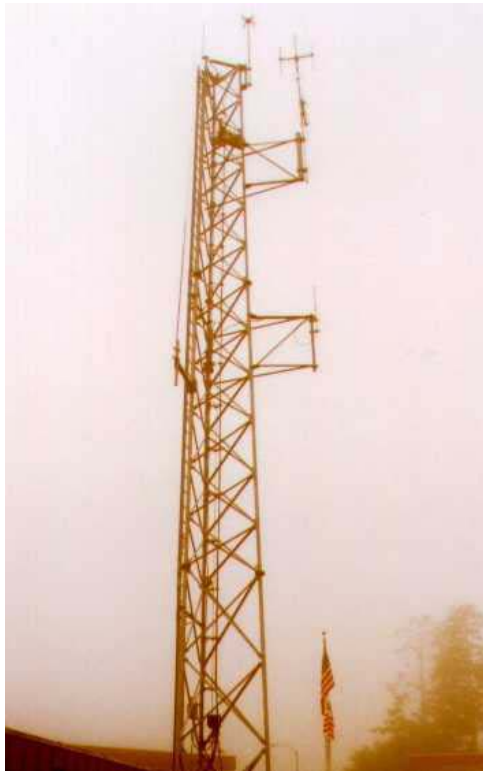
Figure 1-4 60ft Self supporting communications tower.
