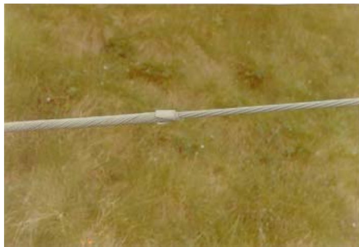
Figure 6-3 End sleeve installed on guy-grip dead end.
