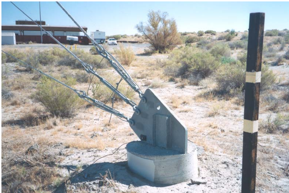
Figure 6-5 Structural guy anchor on a 625ft Loran-C tower.
