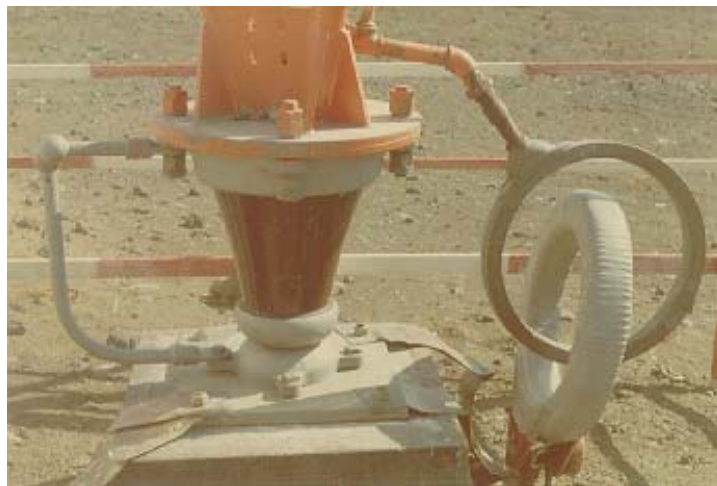
Figure 5-3 Cone shaped base insulator.
