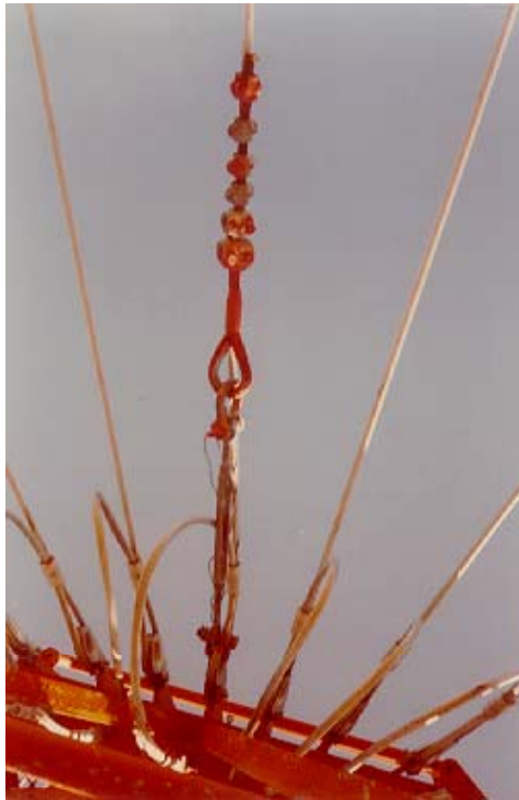
Figure 6-4 "Sister Wire" consisting of shackles, turnbuckles, wire rope segment with preformed eye, reinforcing a TLE on a Loran tower.
