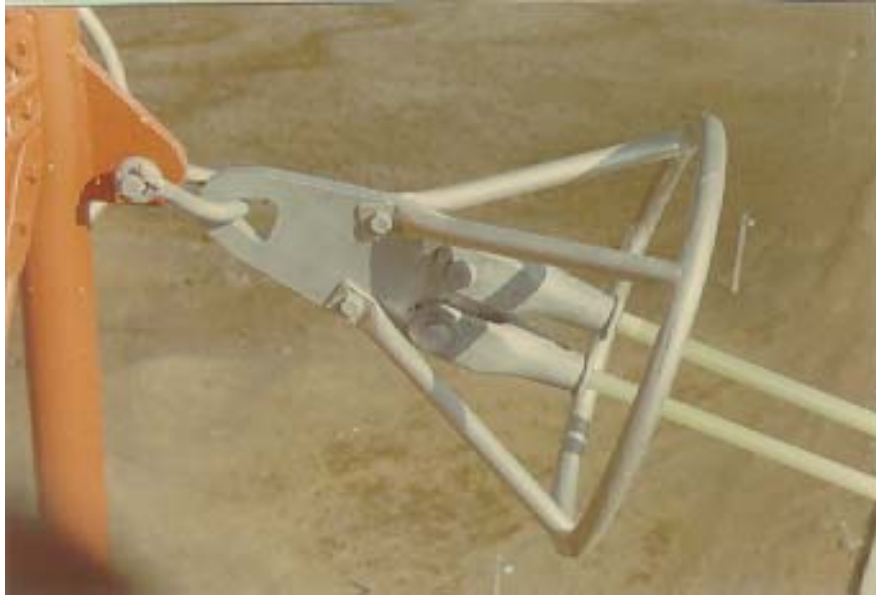
Figure 6-12 One type of corona ring, in place on a structural guy.
