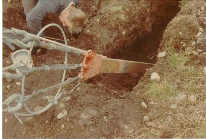
Figure 4-1 Excavation and inspection around anchor arm.
