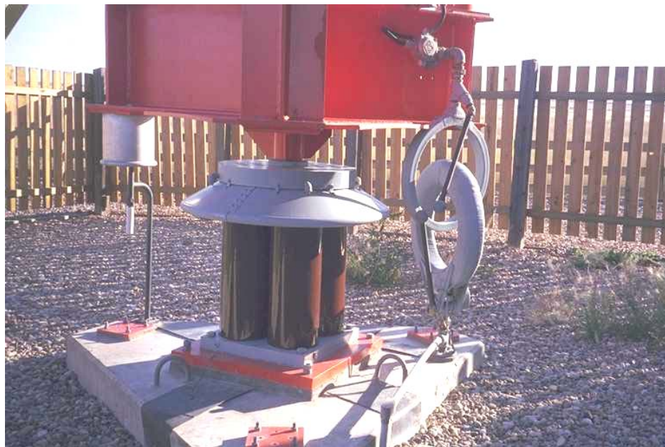
Figure 5-6 Oil-filled multiple cylinder base insulator.
