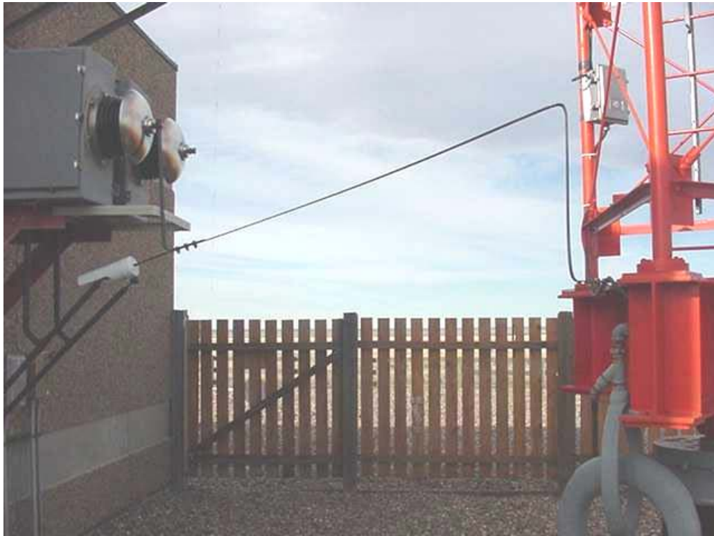
Figure 9-4 Typical "z-feed" used at a LORAN Station.
