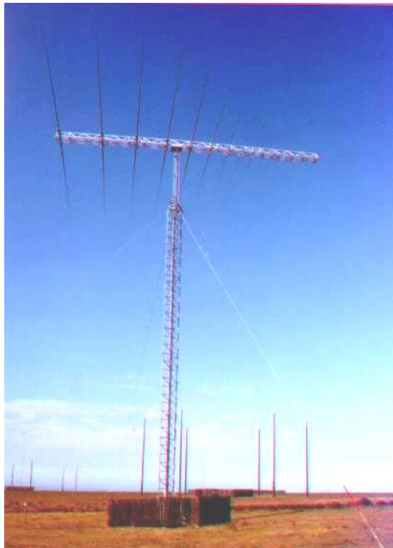
Figure 1-5 Guyed rotatable antenna
