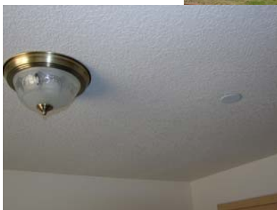
(inset) shows an installed fire sprinkler with flush mounted ceiling cover, far right in photo, in one of the new homes in Carlton's Rolling Hills subdivision (above).
