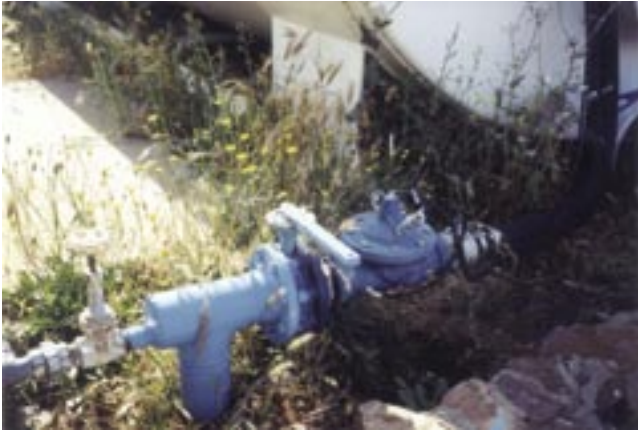
Figure 56—Automatic water valve.
