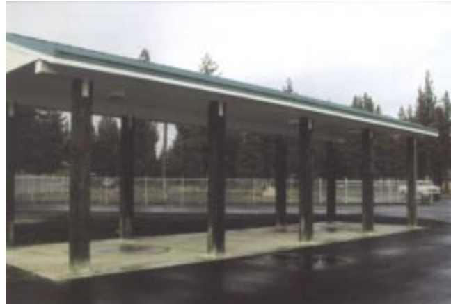
Figure 25—Retardant storage structure.
