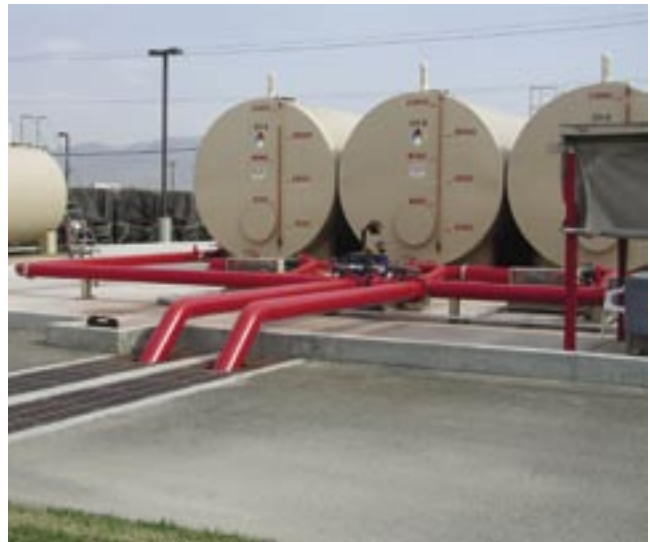
Figure 38—Mixing and storage area night lighting (San Bernardino, CA).
