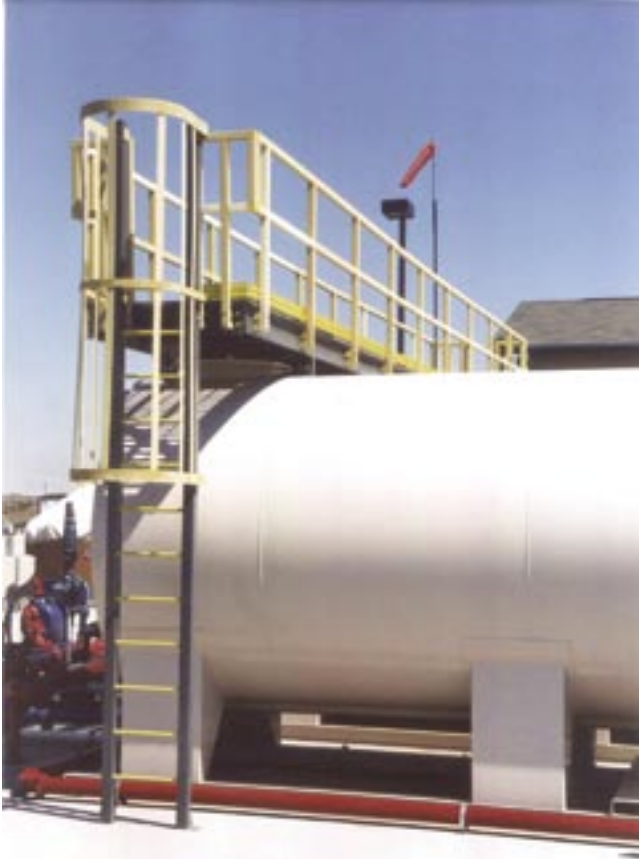
Figure 36—Platform over tanks (JEFFCO, CO).
