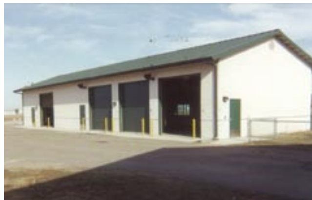
Figure 66—Storage building with contractor work and storage area included (Porterville, CA).
