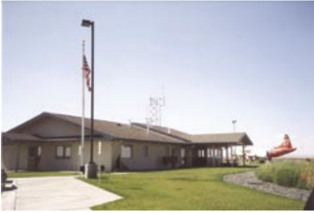
Figure 67—Retardant base operations office (Moses Lake, WA).
