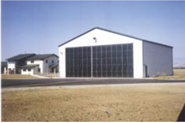
Figure 26—Hangar (Porterville, CA).
