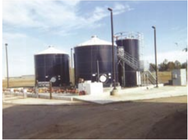
Figure 37—Stairway and ladder to overhead decks (Porterville, CA).
