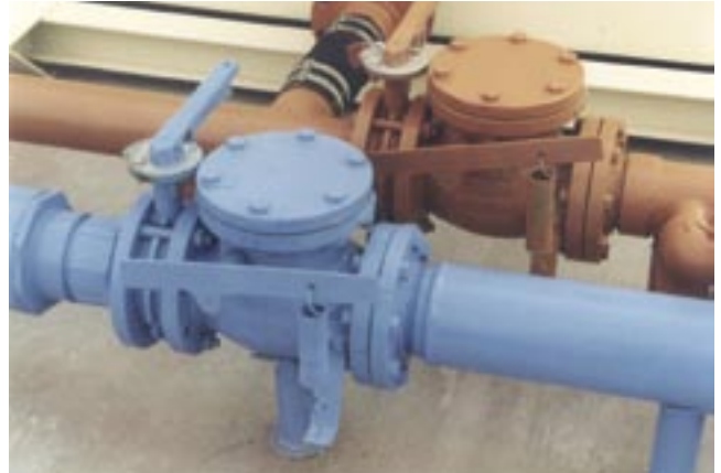
Figure 47—Check valves.
