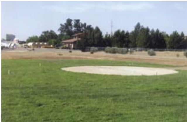
Figure 33—Example of a well-turfed heliport.
