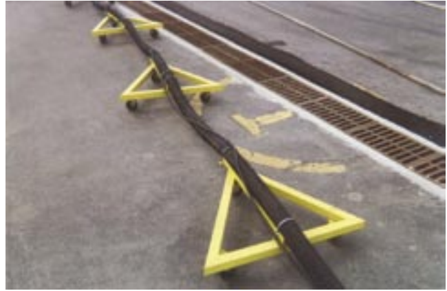
Figure 61—Loading hose and hose skates (JEFFCO, CO).
