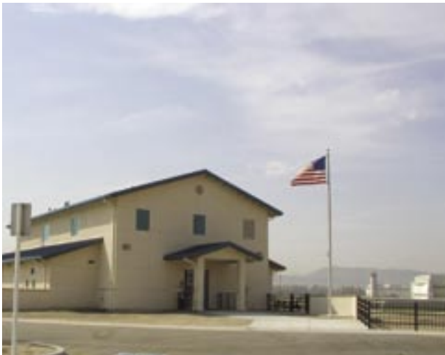
Figure 18—Retardant base operations building (San Bernardino, CA).
