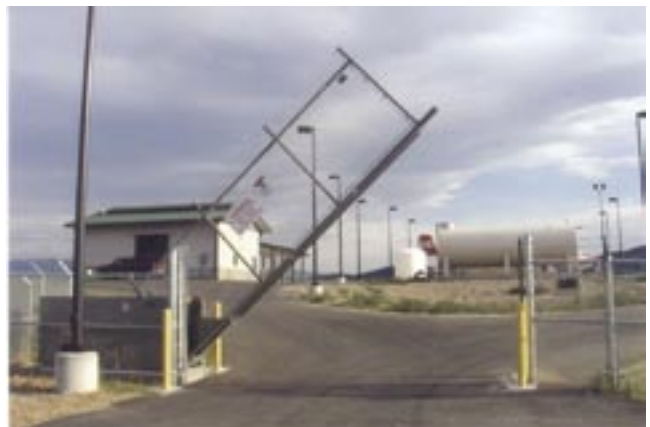
Figure 76—Base fencing and security gate (Helena, MT).
