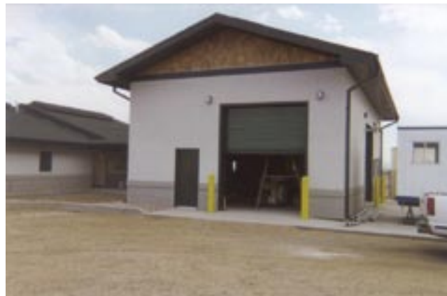
Figure 65—Storage building (JEFFCO, CO).
