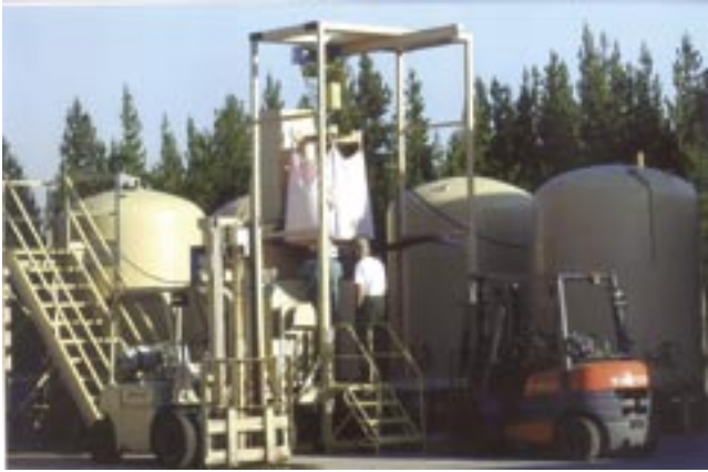
Figure 40—Automatic dry powder batch mixer (12) (West Yellowstone, MT).
