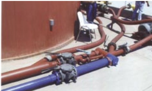
Figure 44—Inline proportioner, orifice blender (Redmond, OR).
