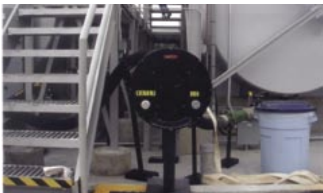
Figure 46—Inline proportioner, Vari-blender (McCall, ID).
