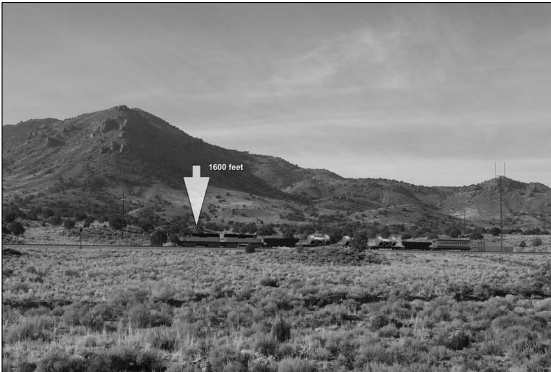
Figure D-60. Simulation of train in view south-southwest from key observation point 23. Note simulation of signal in left midground, communications tower in right midground. Power poles are not simulations.
