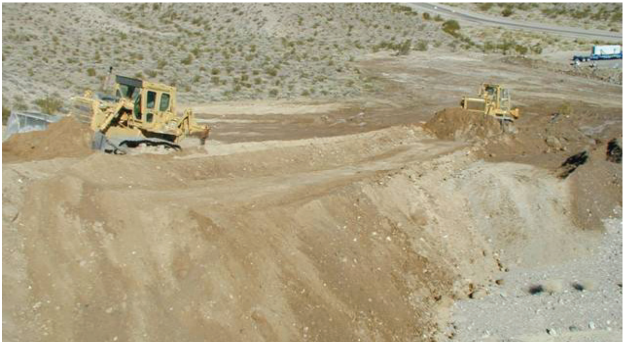
Figure 4-2. Fill material is spread and contoured on the site of a decommissioned borrow area.
