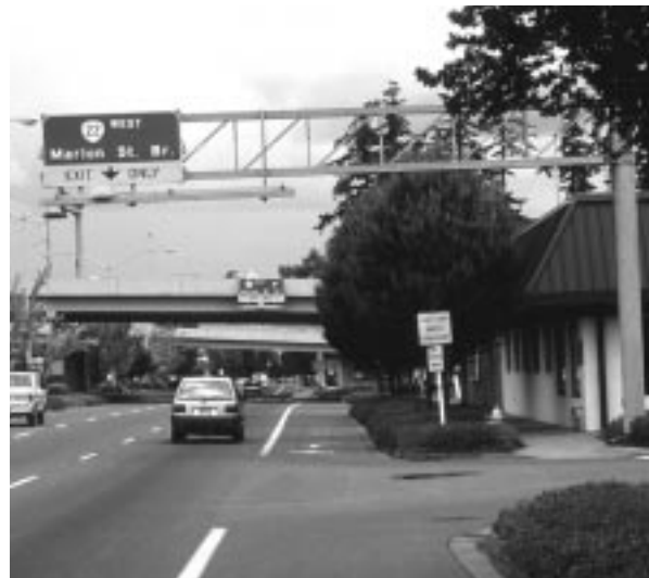
Directional signs placed high are not visible to pedestrians
