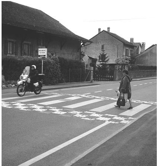
Raised and textured crosswalk (Switzerland)
