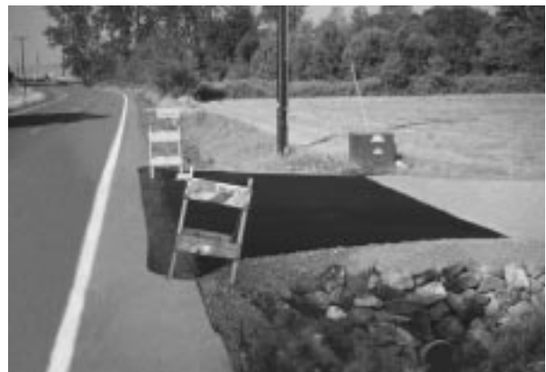
Gravel driveway with paved apron
