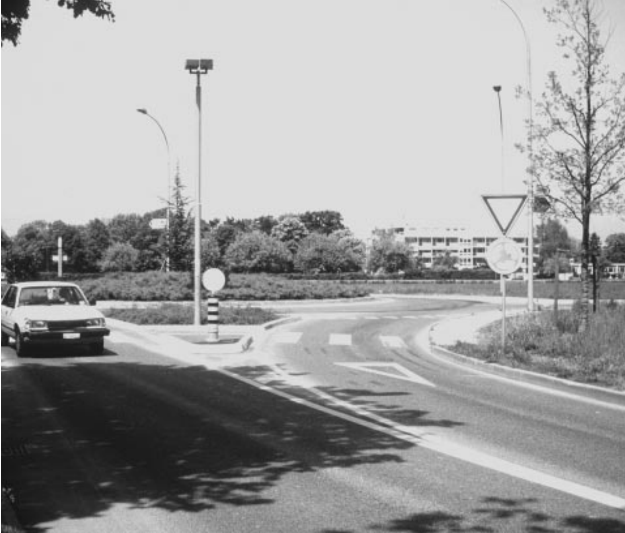
Modern roundabout (Switzerland)
