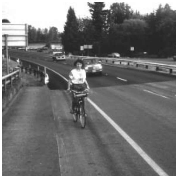
This bridge was restriped to include wider shoulders
