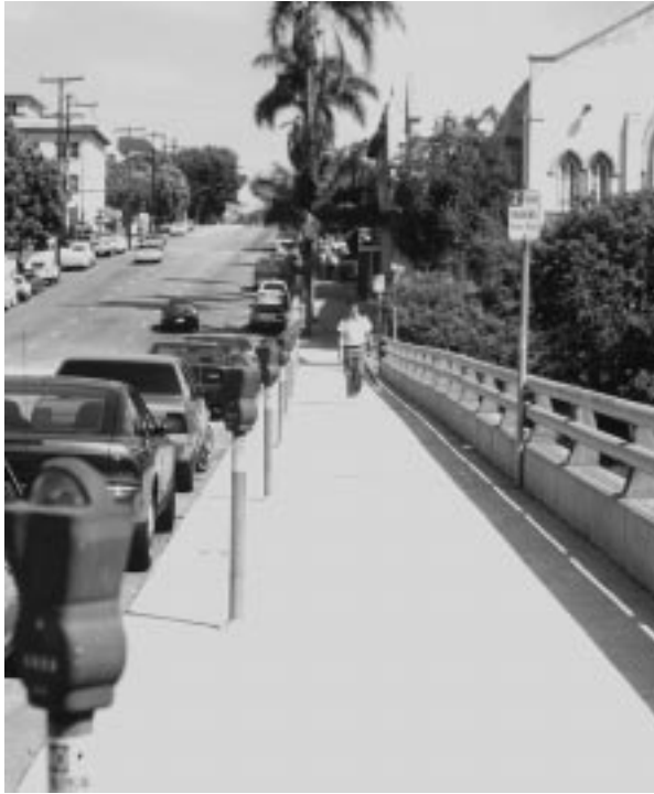
Wide sidewalk on bridge with parking meters
