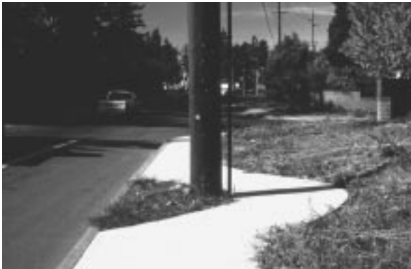
Sidewalk wraps around poles
