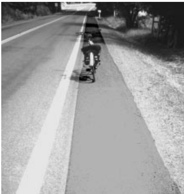
Chip seal leaves adequate shoulder width
