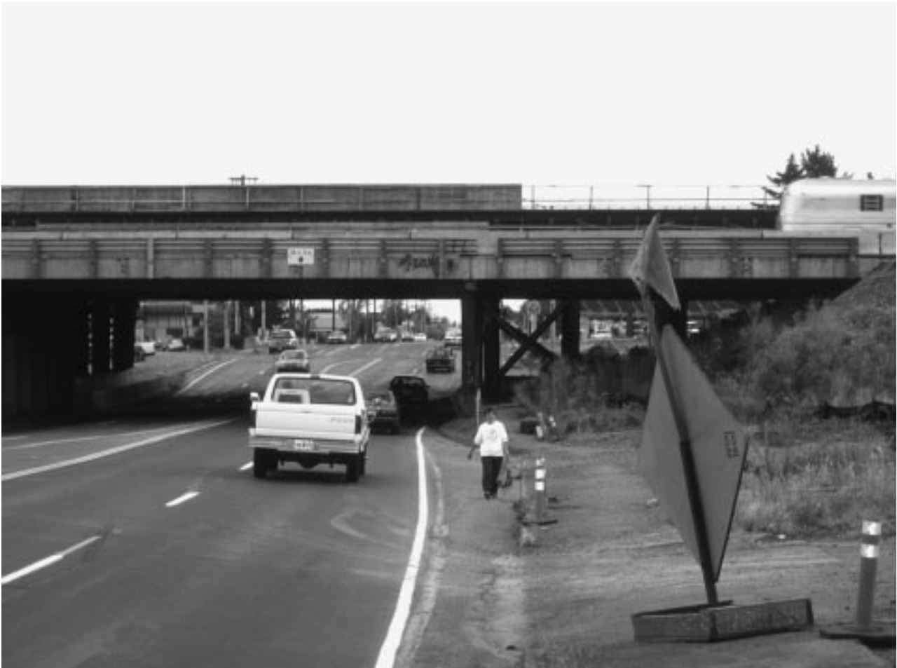
Pedestrians need access across freeway during construction
