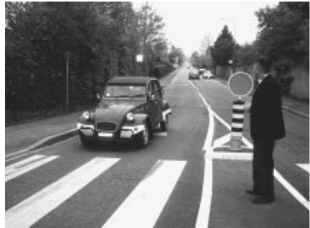
Crosswalk at roundabout approach
