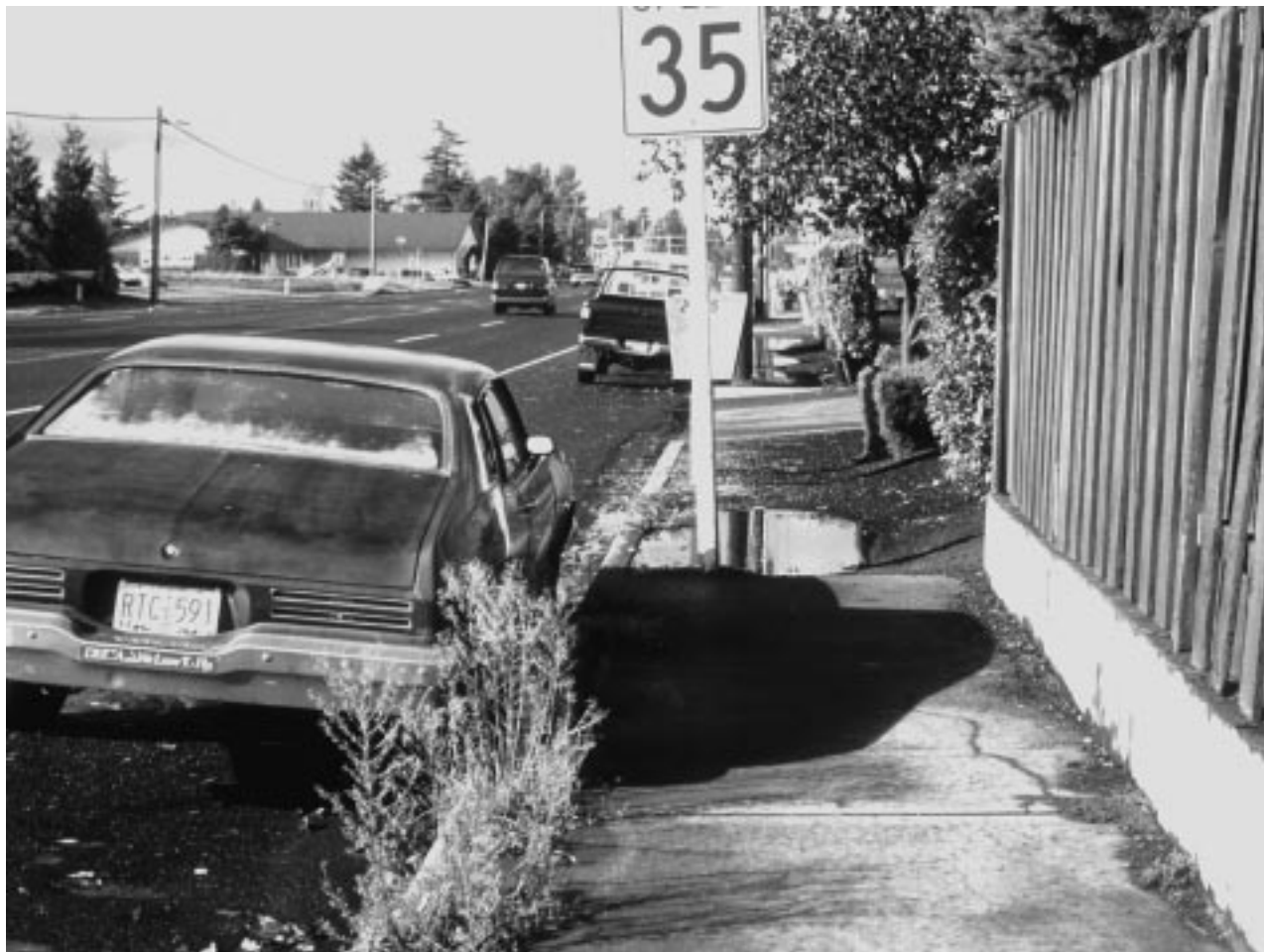
Abandoned driveway should be retrofitted with sidewalk
