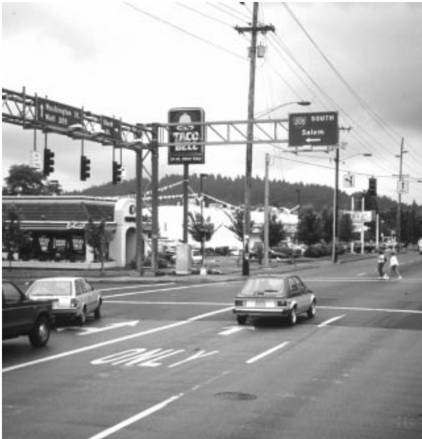
Signals and right-angle intersection make this freeway entrance crossable by pedestrians
