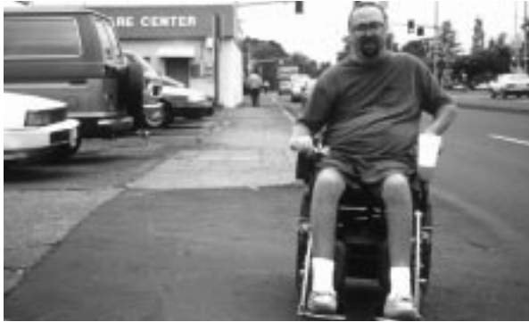
Steep cross-slope tilts wheelchair
