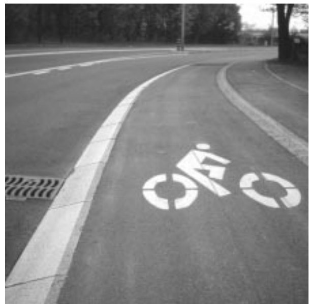
Raised bike lane
