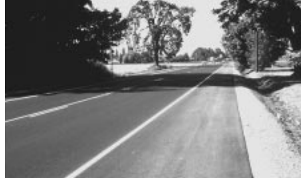
This overlay project added smooth, paved shoulders
