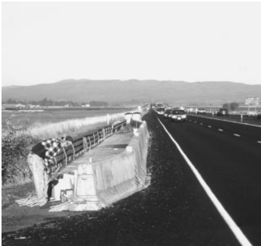
Rural highway construction project with sufficient shoulder width maintained
