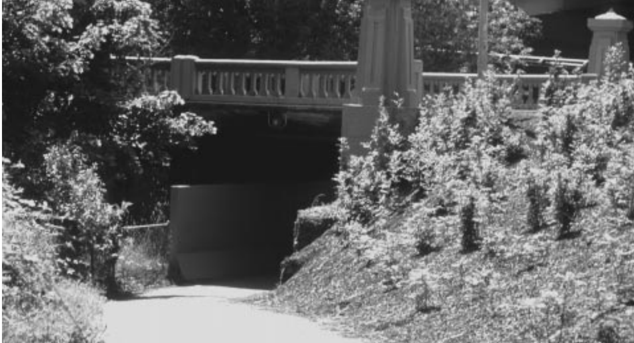
Encroaching vegetation and poor sight distance create an undesirable situation
