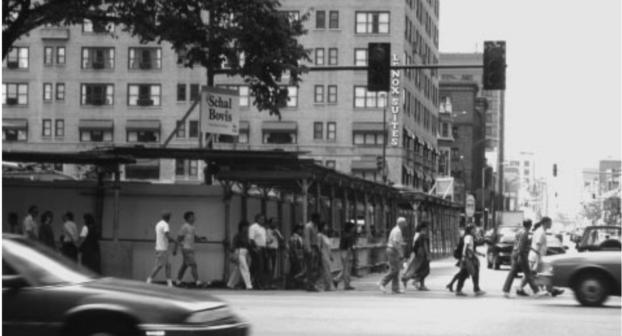
Sidewalk maintained and protected during construction
