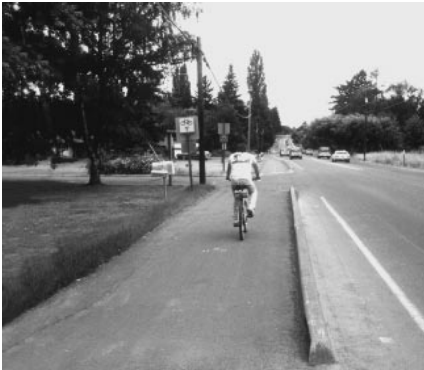
Path adjacent to roadway creates conflicts at intersections
