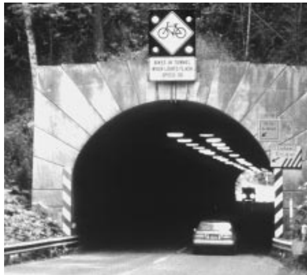
“BIKES IN TUNNEL” sign on the Oregon Coast Highway
