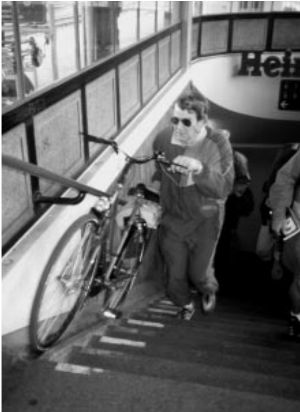
Groove in stairway provides bicycle access to underground passage
