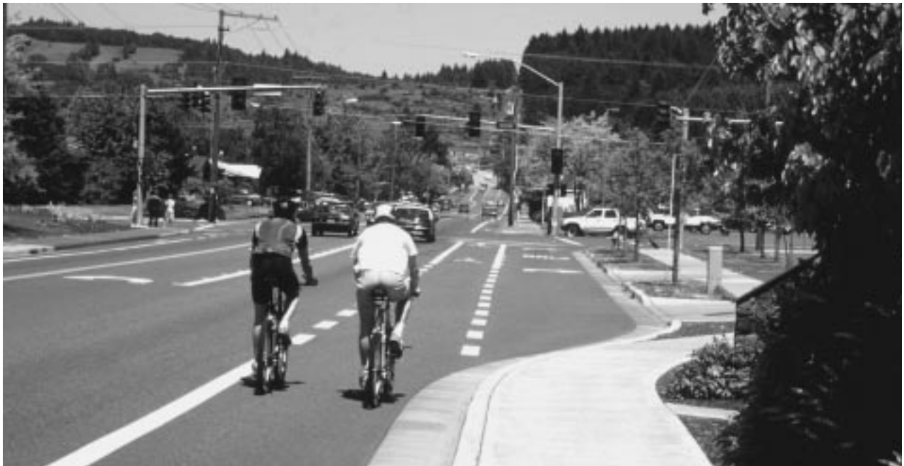
Through bike lane striped to left of right-turn lane
