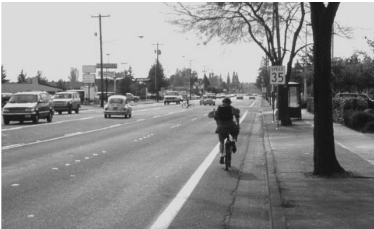
Bike lanes were striped on this arterial by narrowing travel lanes
