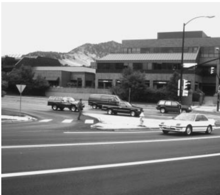
Large island offers protection for pedestrians at this intersection
