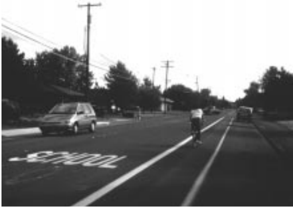
Parking was removed from one side to provide bike lanes
