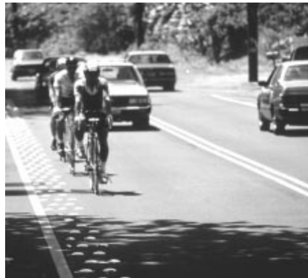
Raised reflectors force cyclists into travel lane
