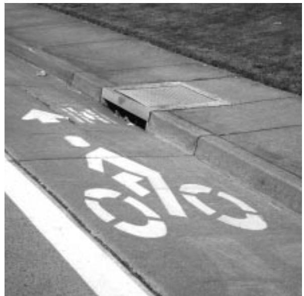
Inlet in the curb face
