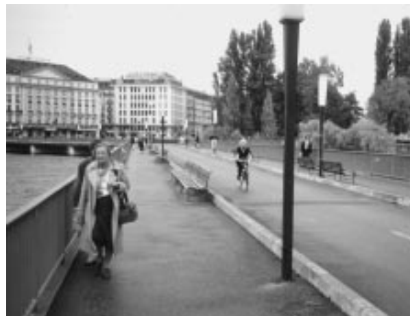
Wide pedestrian and bicycle bridge
