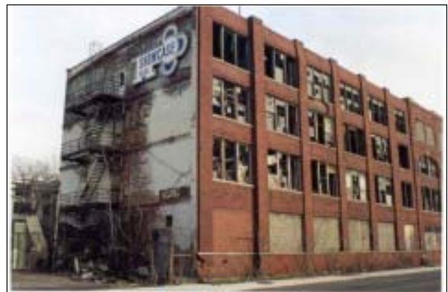
Figure 1. Figure 98. Brownfield site in Detroit, Michigan, 1998.
