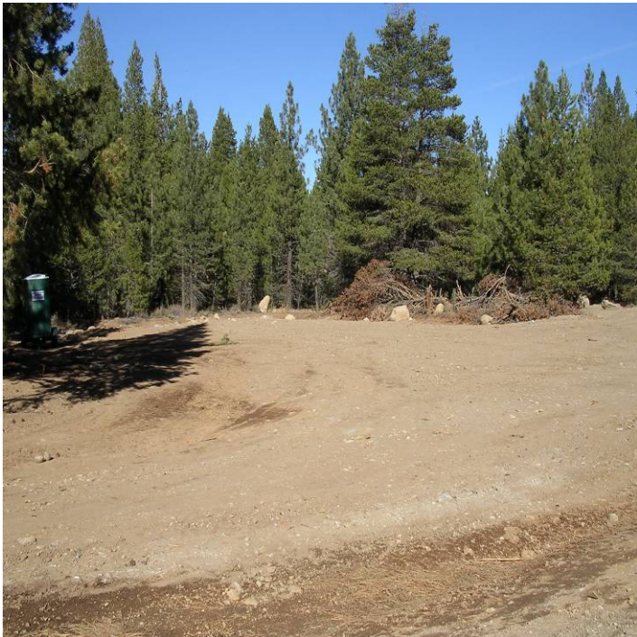
Figure 1. The lead contaminated topsoil has been removed during the summer of 2007.
