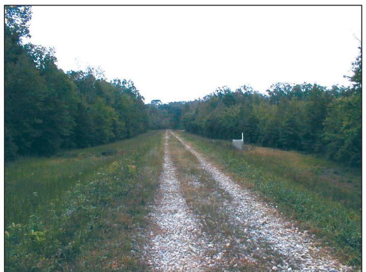
Figure B1. Photographs showing vegetation and topography of (A) the Sinking Pond spillway and the constructed berms at (B) Westall Swamp and (C) Huckleberry Creek.
